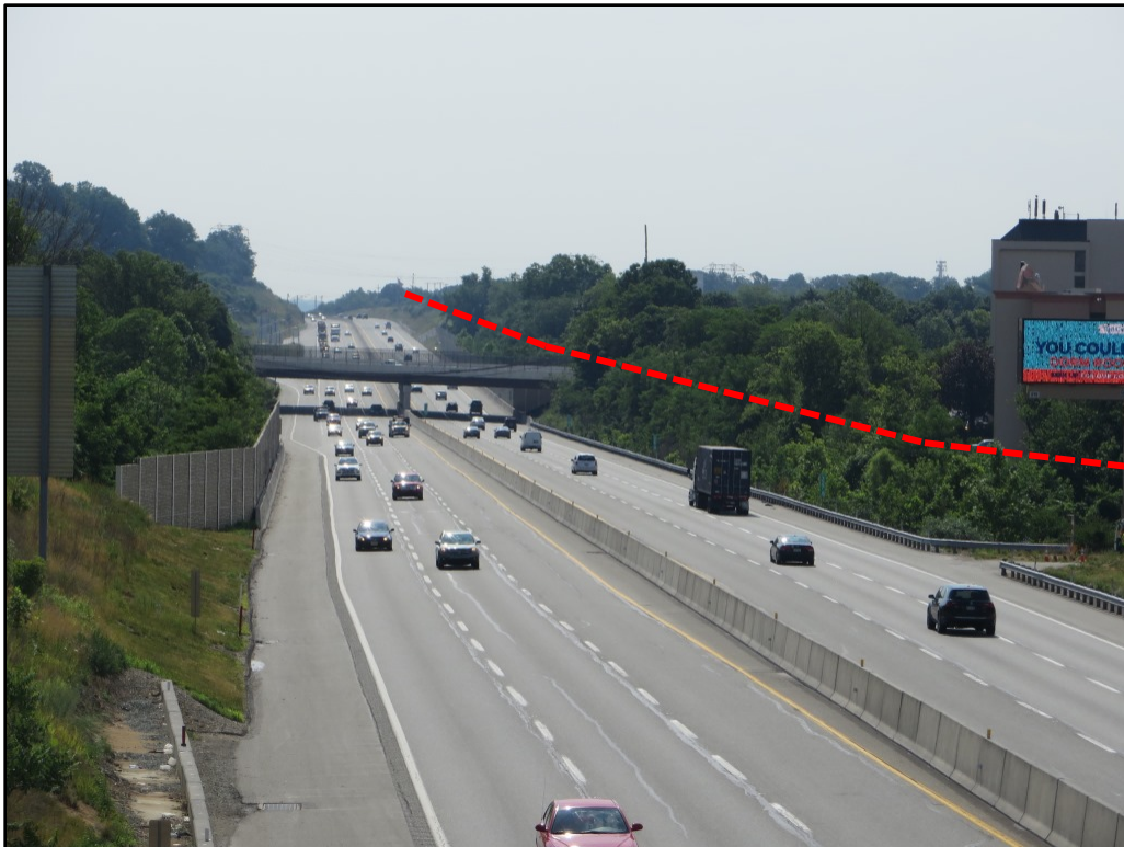
Photograph 4. Pennsylvania Turnpike, view to southeast from Allendale Road bridge, showing proposed KOP Rail Project elevated track location.
