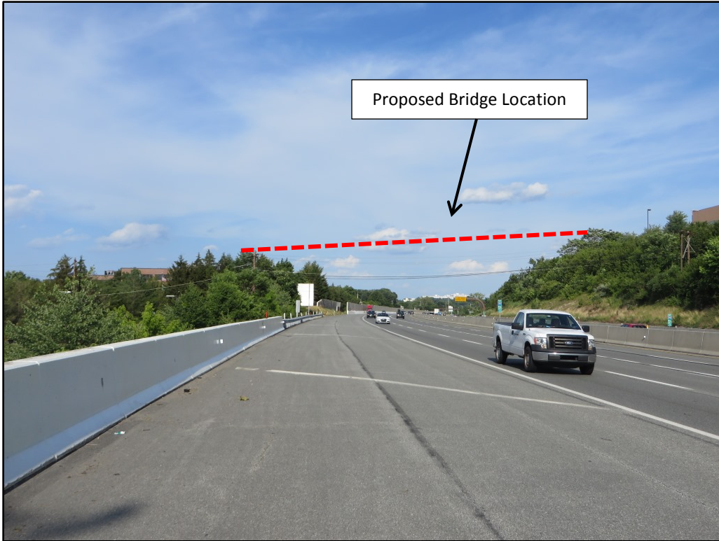
Photograph 5. Pennsylvania Turnpike, view to northeast toward proposed west bridge crossing location at MP 327.
