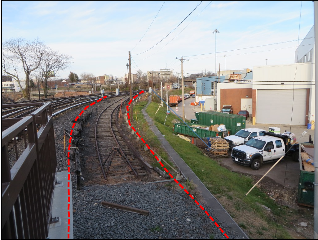
Photograph 13. View looking west along the proposed new track location on the northwest side of the 69 th Street Transportation Center; existing NHSL tracks are at left.
