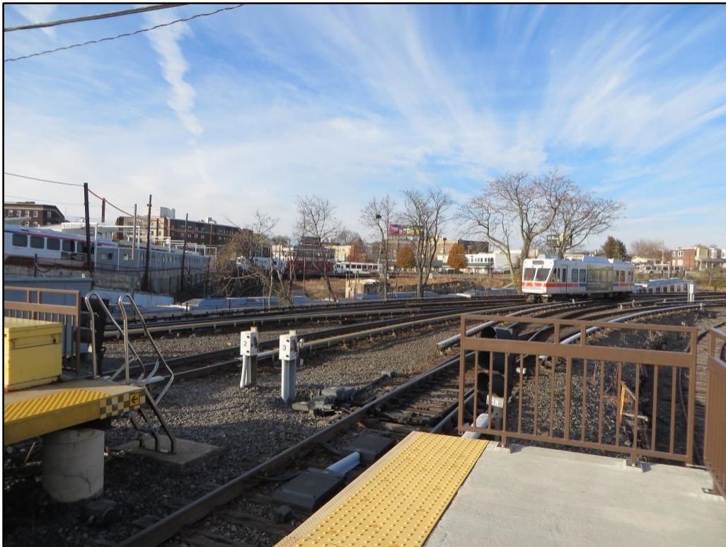
Photograph 10. Philadelphia & Western Railway; Norristown High Speed Line in Upper Darby Township, Delaware County; trackbed view to west from 69 th Street Transportation Center.
