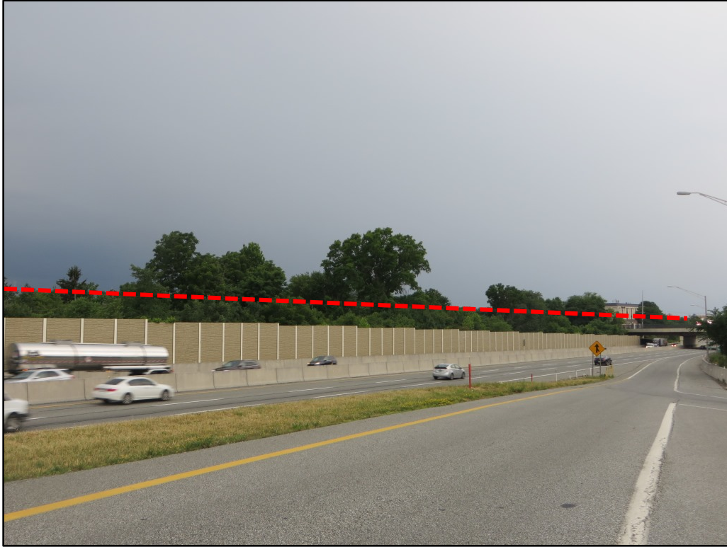
Photograph 3. Pennsylvania Turnpike, view to southwest from King of Prussia Service Plaza, showing proposed KOP Rail Project elevated track location.
