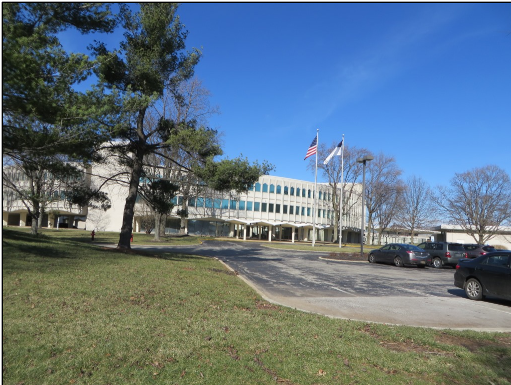
Photograph 6. View looking northeast toward the south entrance of the ABCUSA Mission Center.
