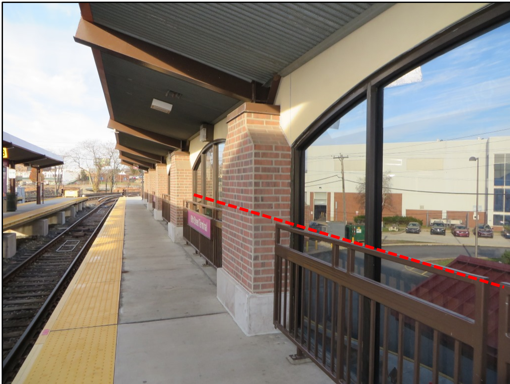
Photograph 14. View looking west along existing north platform at the 69 th Street Transportation Center. New track would be at right; this platform would be widened and the glass wall would be removed.
