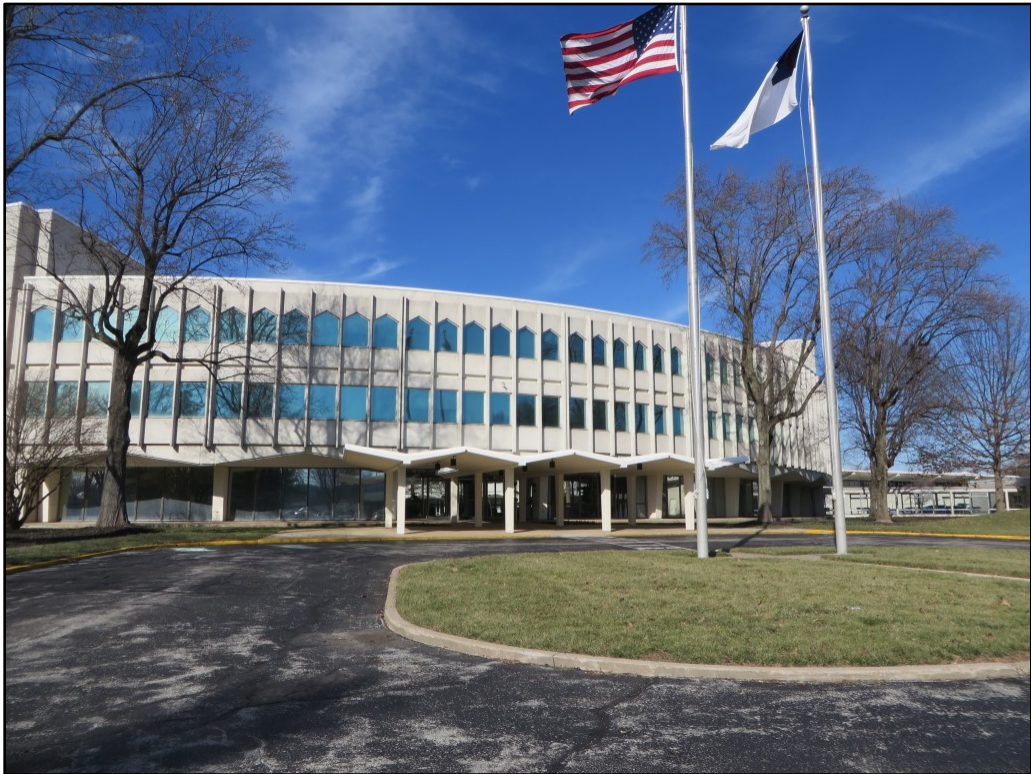
Photograph 12. View of the main south entrance and flagpole circle of the Office and Conference Center, looking northeast.
