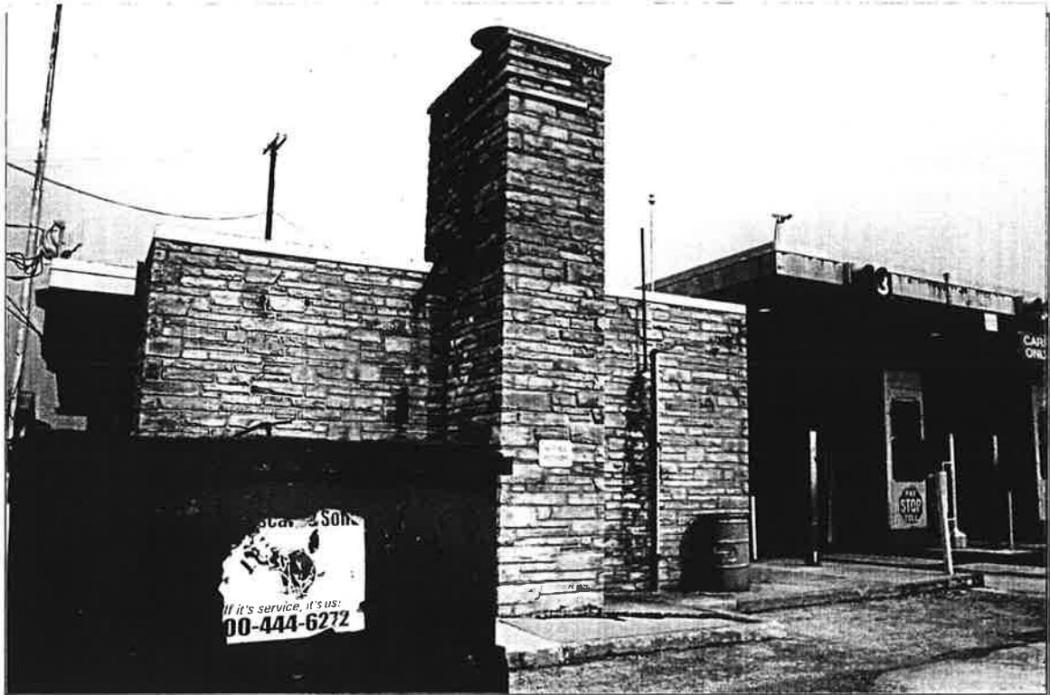
Photograph 3. West elevation, facing southeast.
