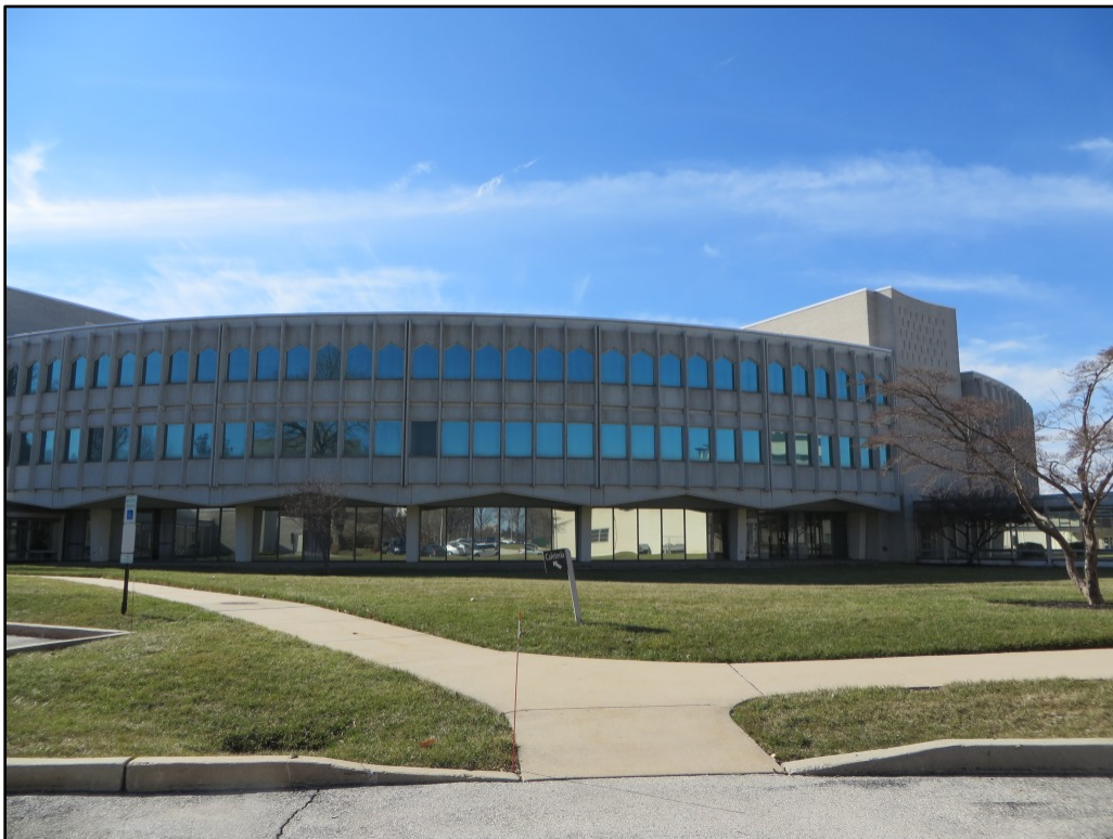
Photograph 14. View looking west toward the east exterior elevation of the Office and Conference Center; note reflective glass in the first floor enclosure, and east hyphen at right.
