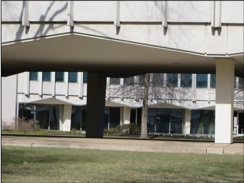
Photograph 17. Circular inner courtyard and inner elevation of the Office and Conference Center, as viewed looking northeast from the southwest perimeter of the building.
