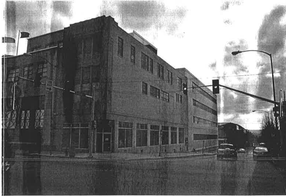
Photograph 6: Former P&W station at the southeast corner of Main and Swede Streets. The trestle formerly ran along the east side of Swede Street to the station.
