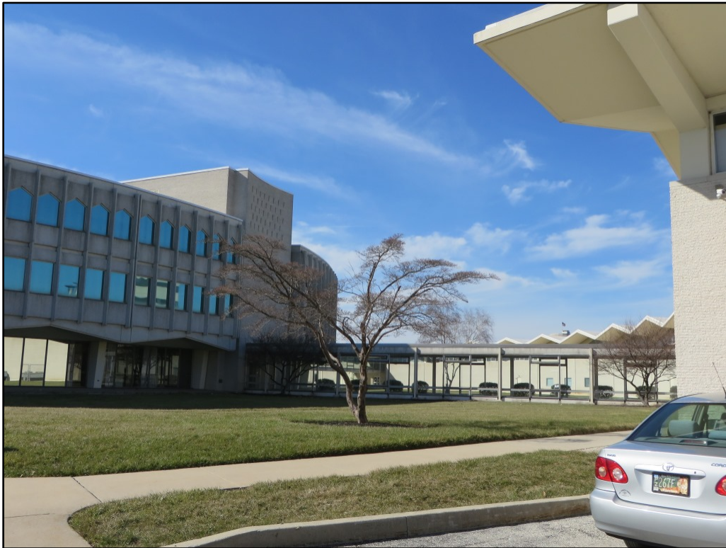
Photograph 30. View looking northwest showing the Office and Conference Center at left and the Graphic Arts Building at right, with east hyphen at center. Behind the hyphen is the inner elevation of the Graphic Arts Building.
