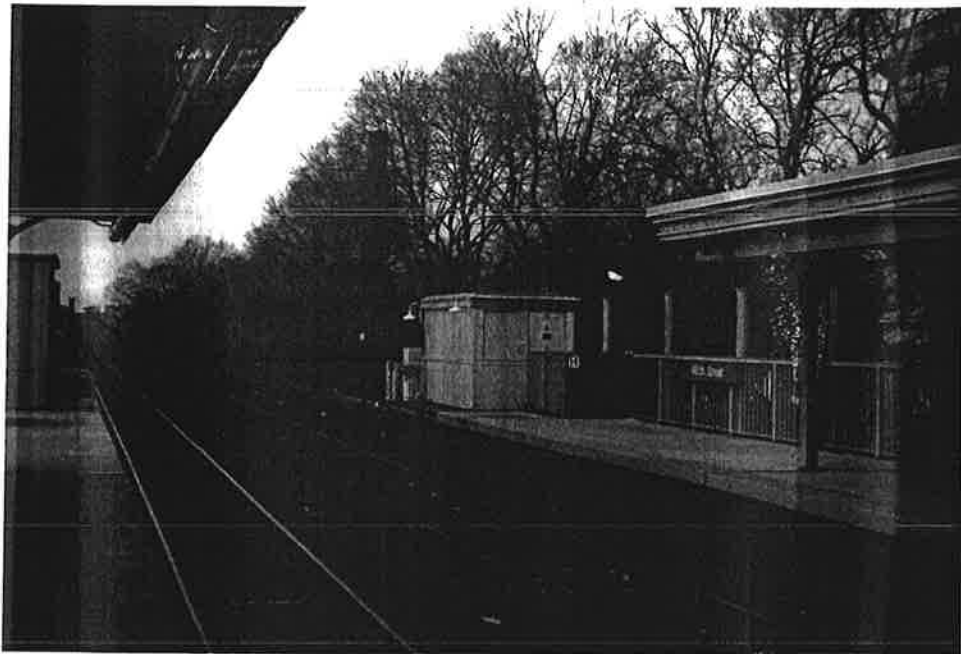
View of historic switching station on eastbound platform of 46th Street Station. Note Classical cornice and paneled facade. Many windows are blocked.
