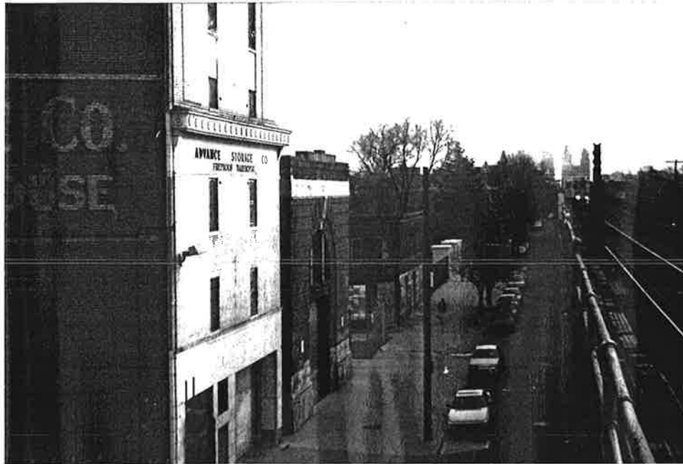
View of Allison Substation looking north from 56th Street Station platform. Note decorative brick pattern and Classical cornice.
