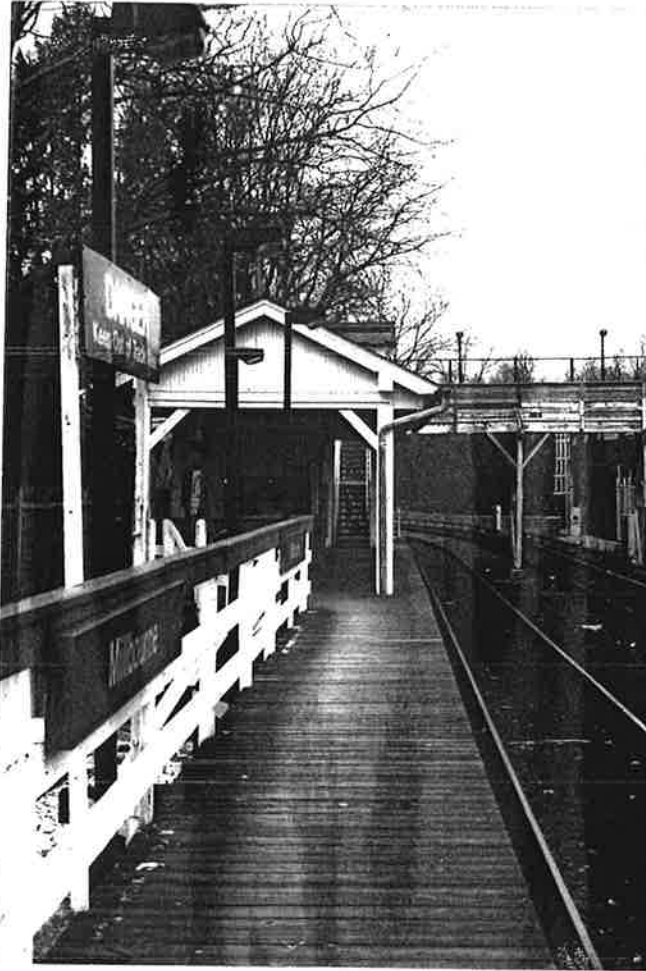
View of eastbound platform looking toward station shelter. Note vertical board in gable-end of shelter. Wood pedestrian bridge located above tracks.
