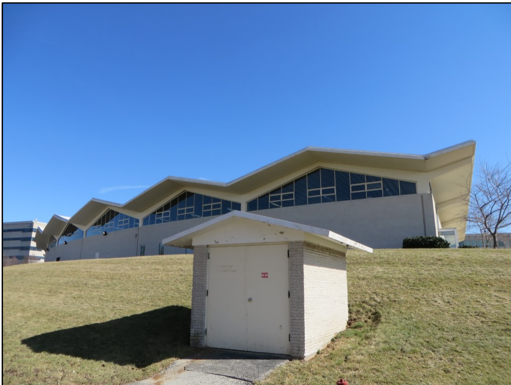
Photograph 32. North (left) and west (right) elevations of the banked utility shed (ca. 1962), located northwest of the Graphic Arts Building; view to southeast.
