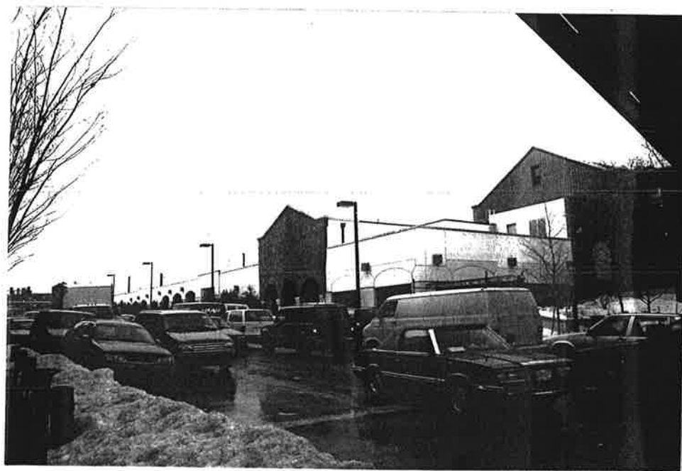
View of reconstructed portion of south facade. Note modern cladding.
