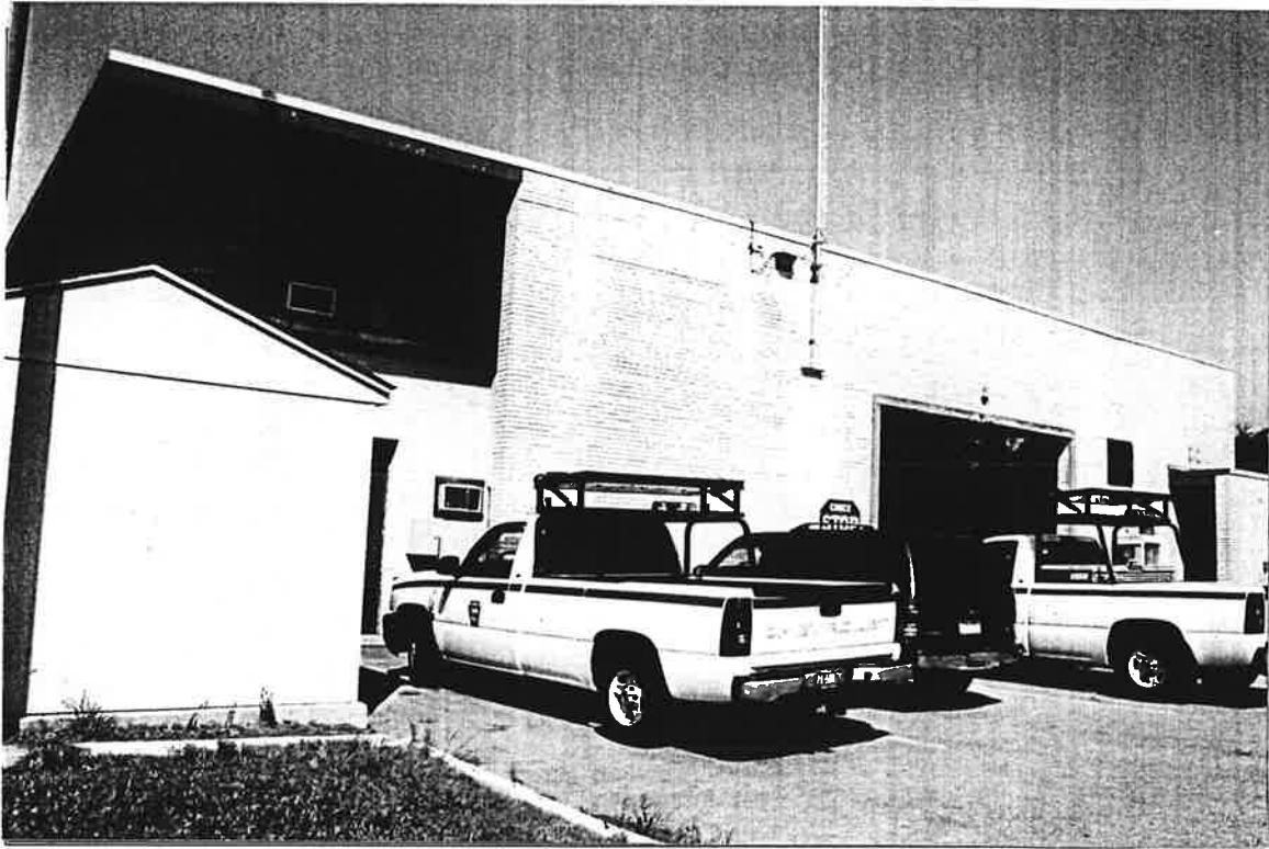
Photograph 2. East elevation, facing northwest.
