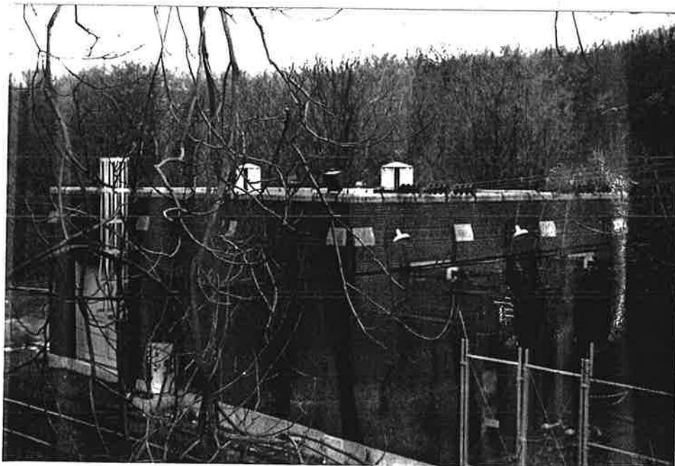
View of brick substation located near westbound tracks. Building was erected circa 1960.
