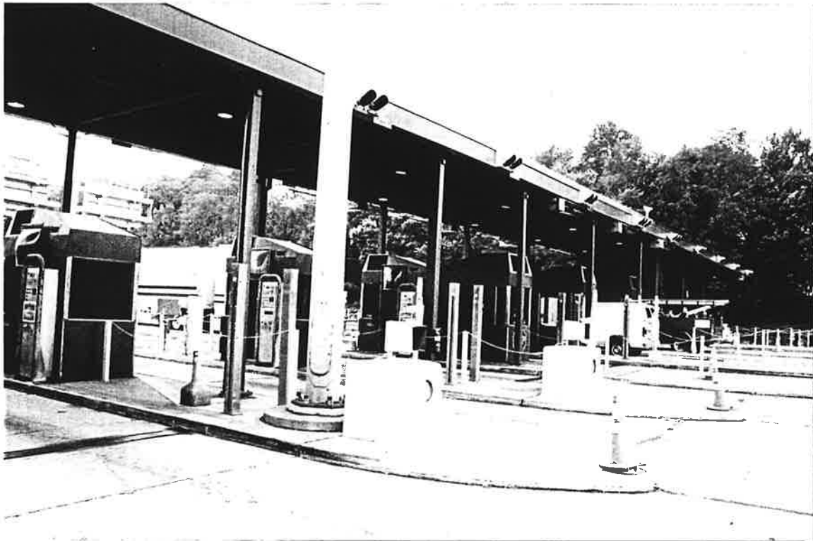
Photograph 5. Detail of tollbooths and canopy, facing north.
