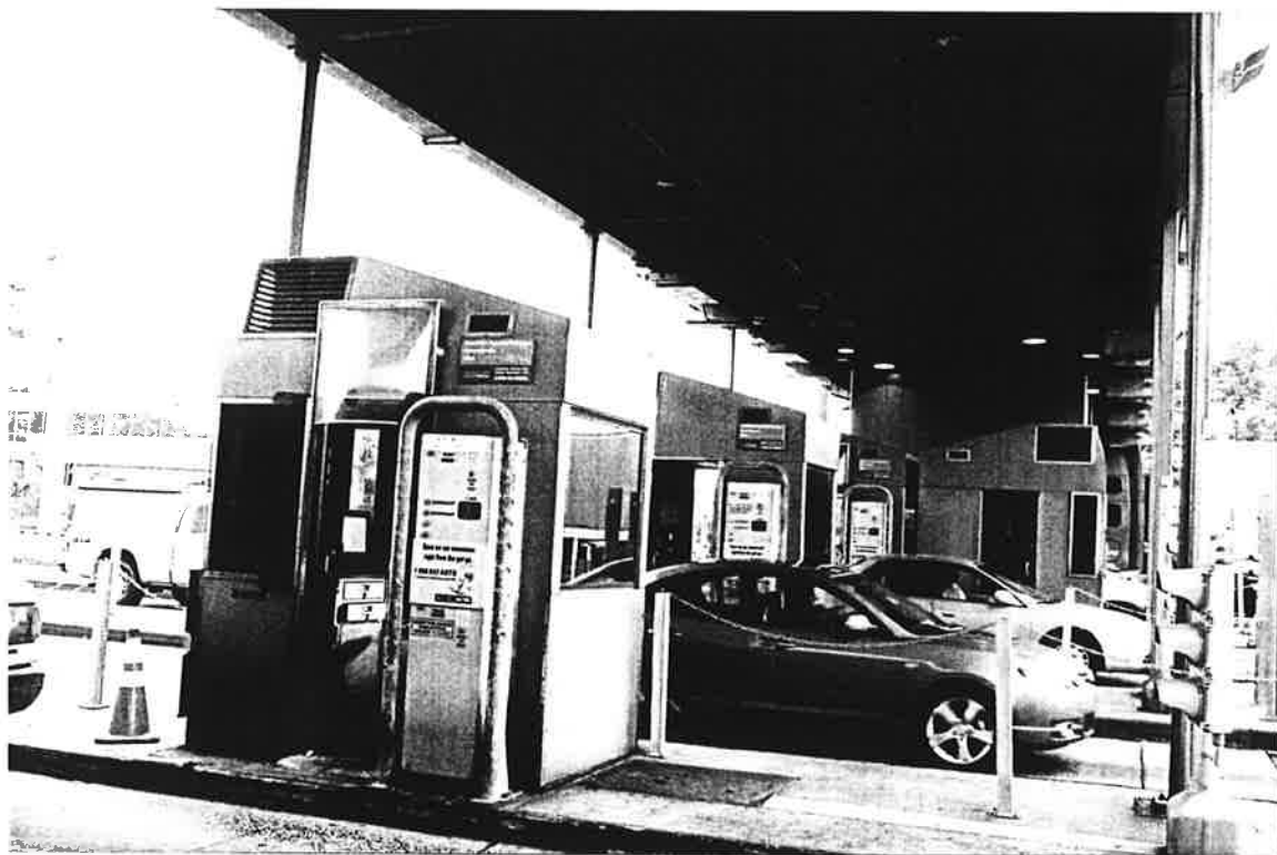
Photograph 5. Detail of tollbooths and canopy, facing northwest.
