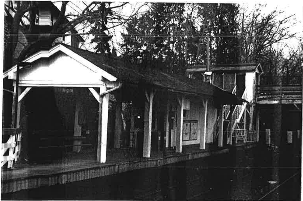
View of eastbound platform at Millbourne Station. Note how bracketed posts support side gable shelter.
