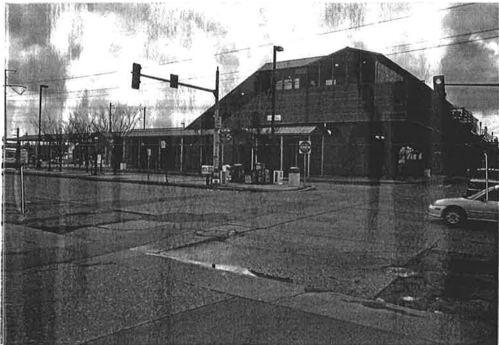
Photograph 5: Norristown Transportation Center with P&W trestle at right in background; taken from the intersection of Lafayette and Swede Streets, facing south.
