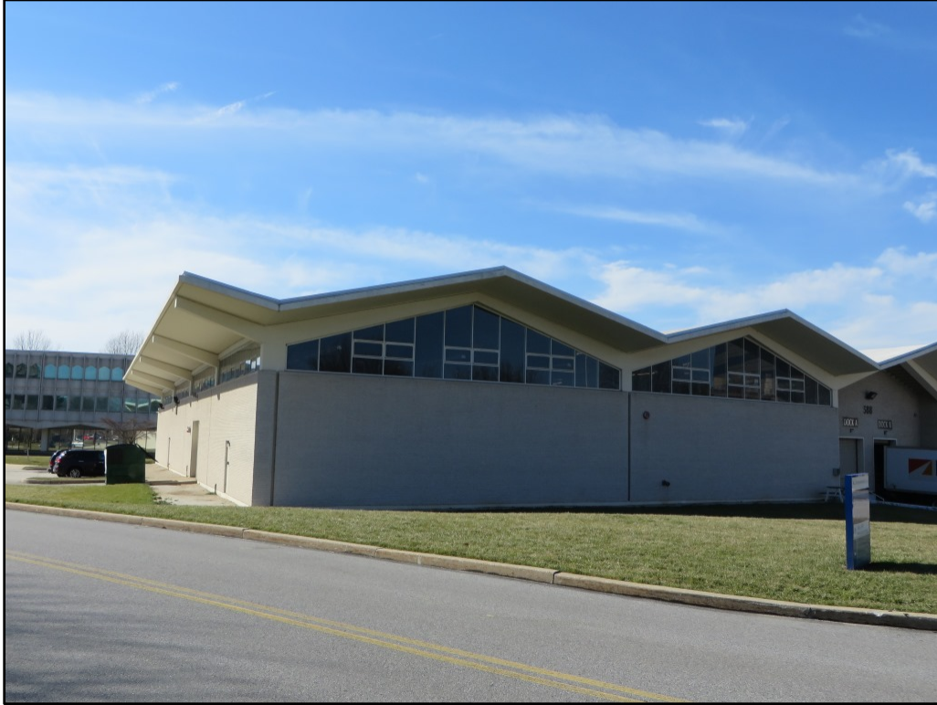
Photograph 29. South elevation (left) and east side of the outer elevation (right) of the Graphic Arts Building, view to west. Second loading dock is at right.
