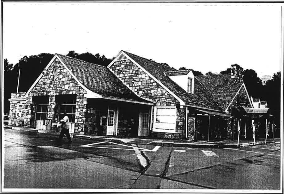
Photograph 2. Southwest corner, facing northeast.
