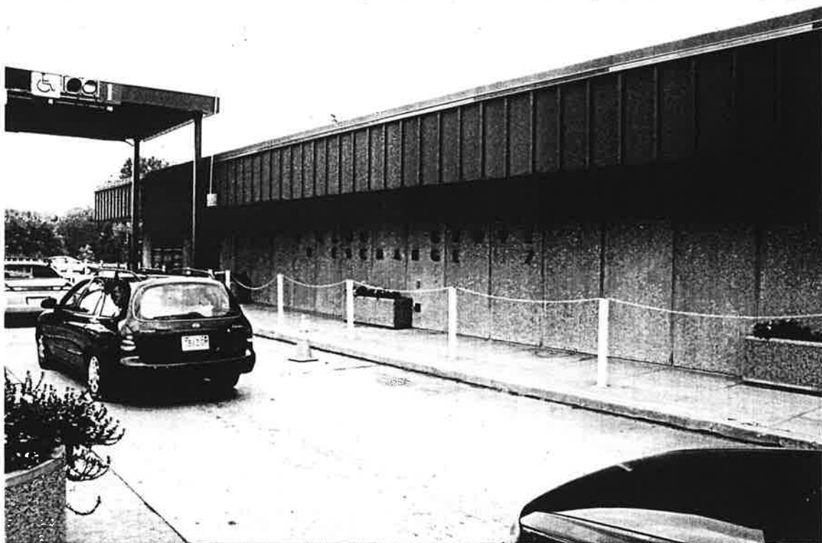
Photograph 2. Northeast elevation, facing south.
