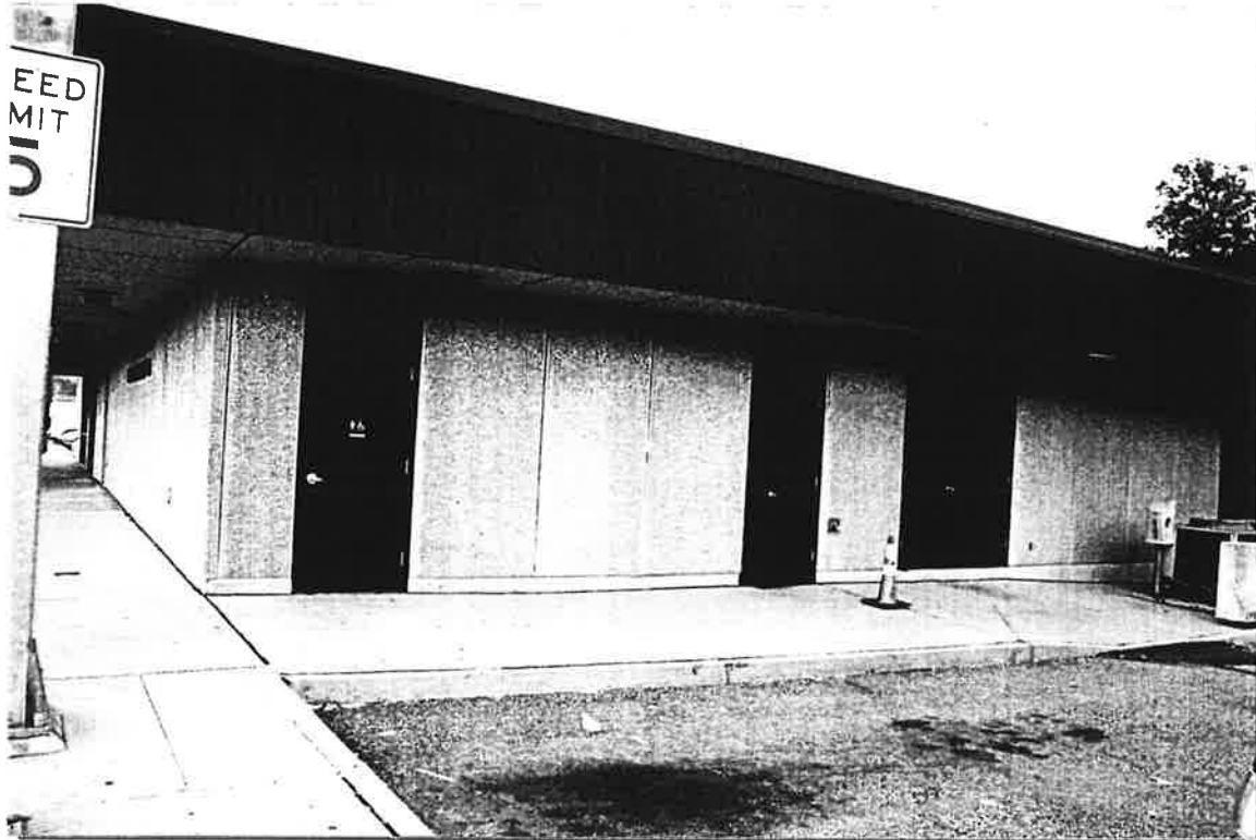
Photograph 2. West elevation, facing southeast.
