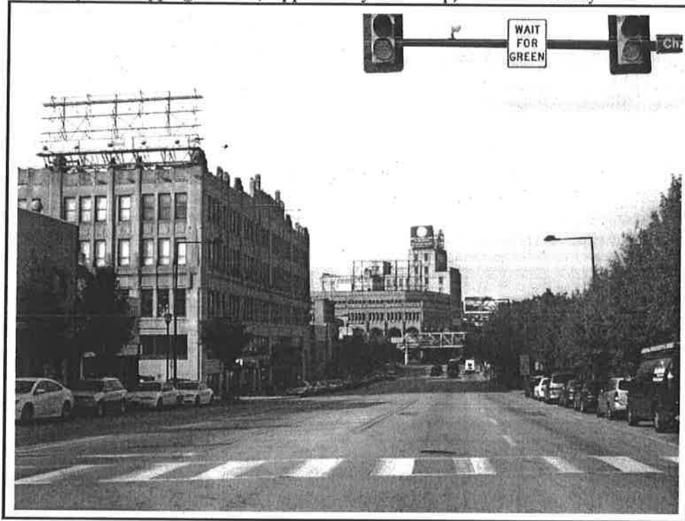
Photograph 6. Overview from the intersection of Chatham Road, showing 6800 Market Street/West Chester Pike on the left, McClatchy Building and former 69th Street Terminal Title & Trust Company in background.
