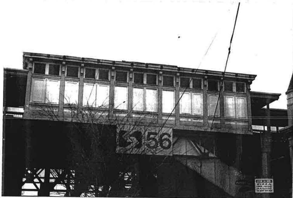
View of exterior of eastbound 56th Street Station. Note Classical copper paneling, pilasters and clerestory windows. Staircases have been reconstructed using modern materials.
