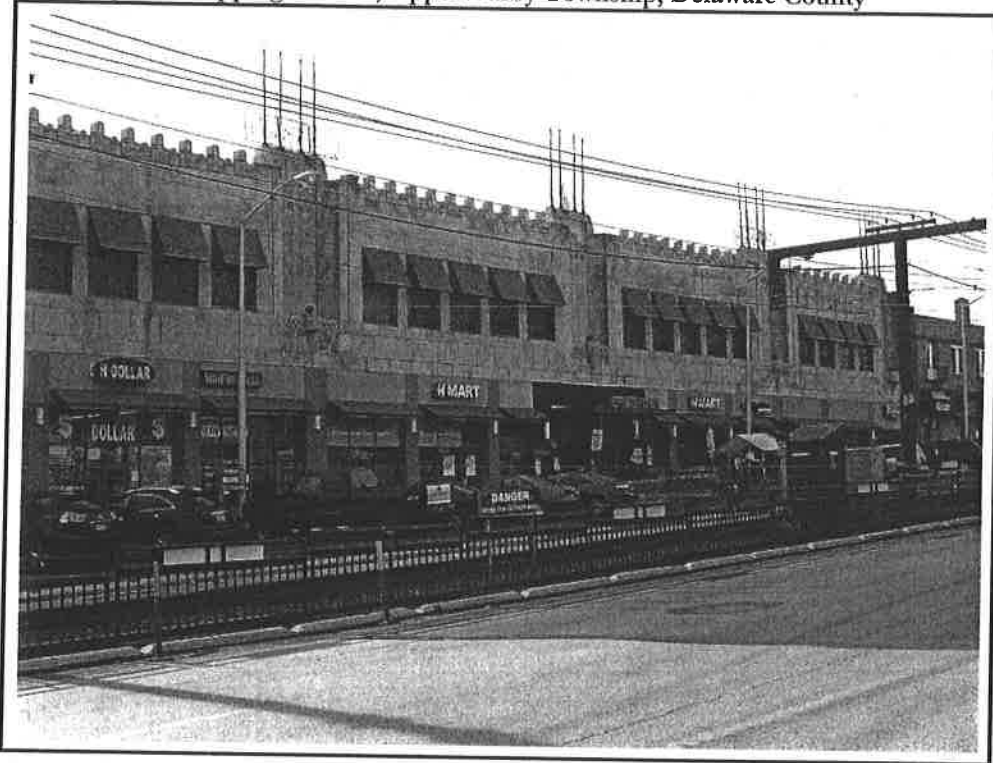
Photograph 21. View of group of commercial buildings showing Art Deco influences with decorative, vertical elements along the roofline.
