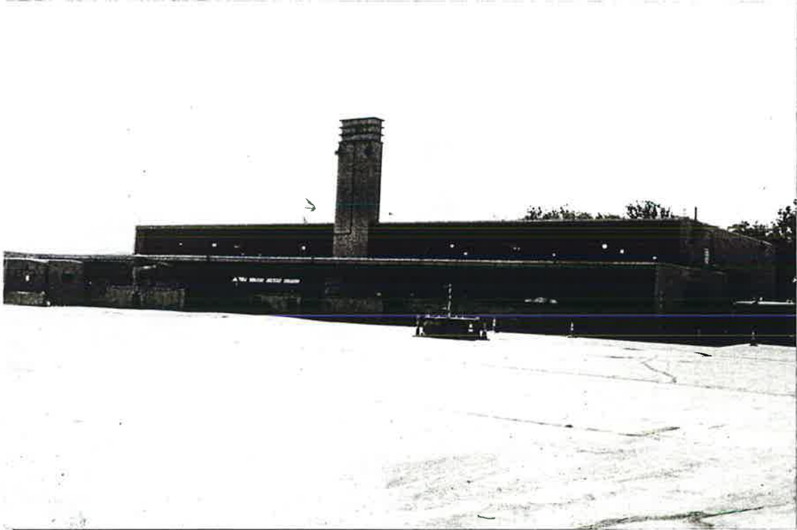
Photograph 3. North (rear) elevation, facing southeast.
