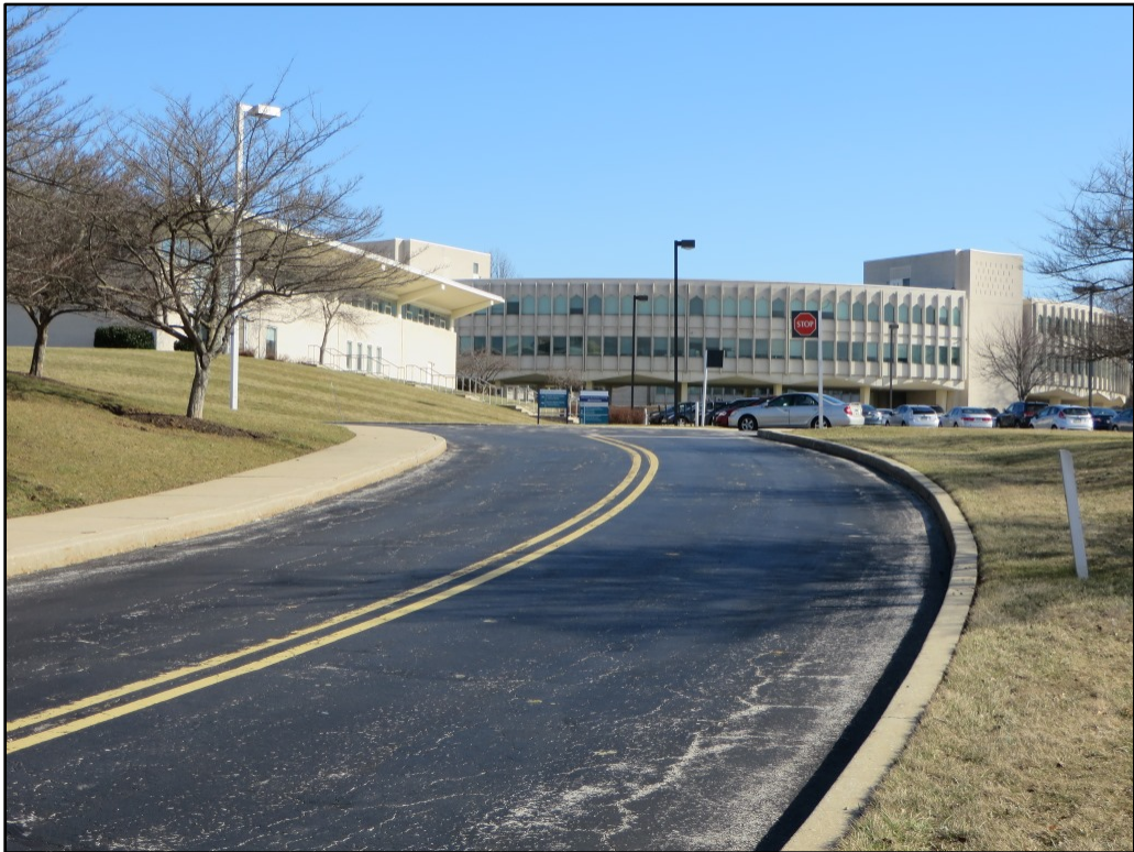
Photograph 6. View looking southeast up the north driveway from 1 st Avenue, showing the Graphic Arts Building at left and the Office and Conference Center at center and right.
