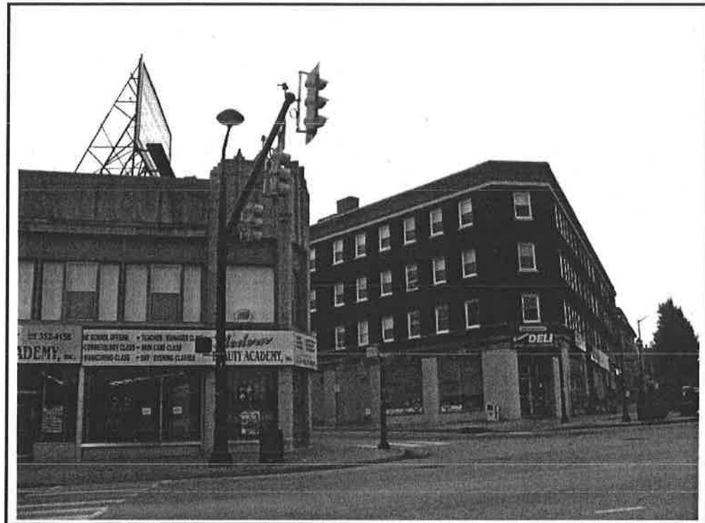
Photograph 18. This shows the intersection of Copley Road and Market Street/West Chester Pike, with the Stonehurst Apartments in the background.
