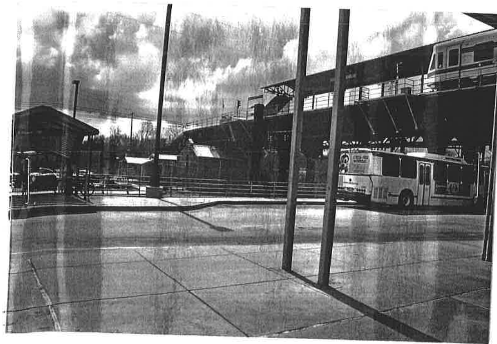
Photograph 9: Norristown Transportation Center, with P&W trestle at right and extending over the buildings in the center of the photograph, facing southwest.
