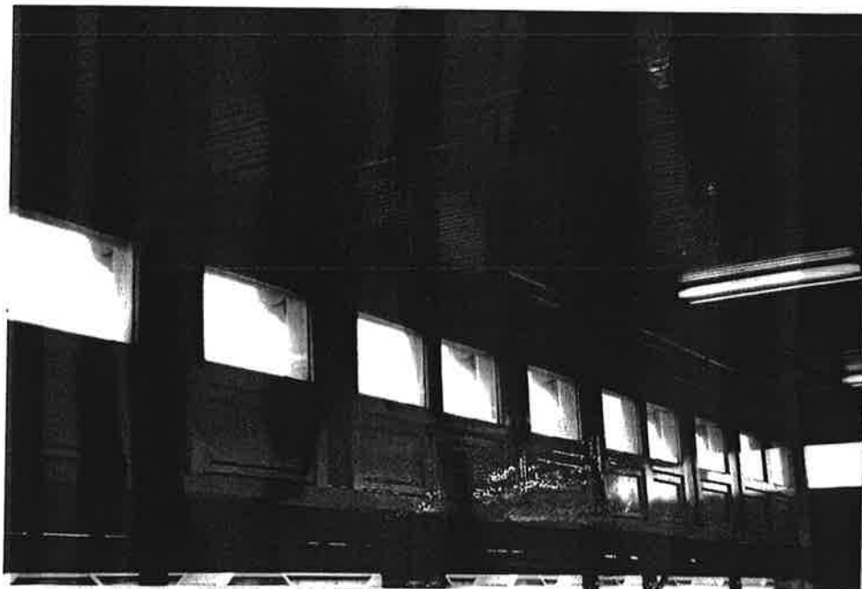
View of interior of westbound 52nd Street Station. Note wood paneling below clerestory windows. Ceiling sheathed in historic wood siding.
