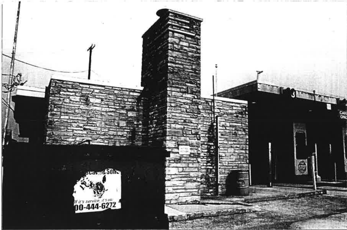
Photograph 3. West elevation, facing southeast.
