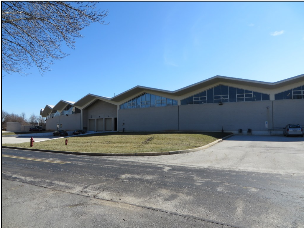
Photograph 28. North side of the outer elevation of the Graphic Arts Building, showing typical fenestration and one of two loading docks, view to southeast.
