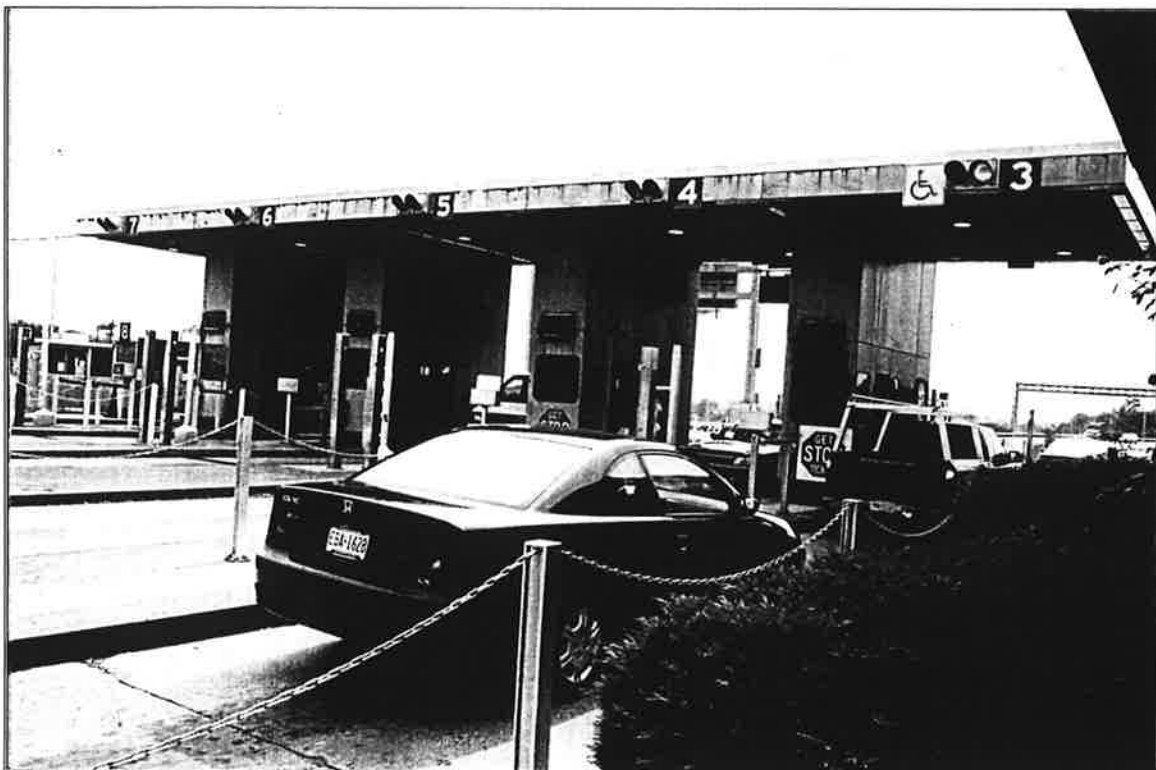
Photograph 4. Detail of tollbooths and canopy, facing southwest.
