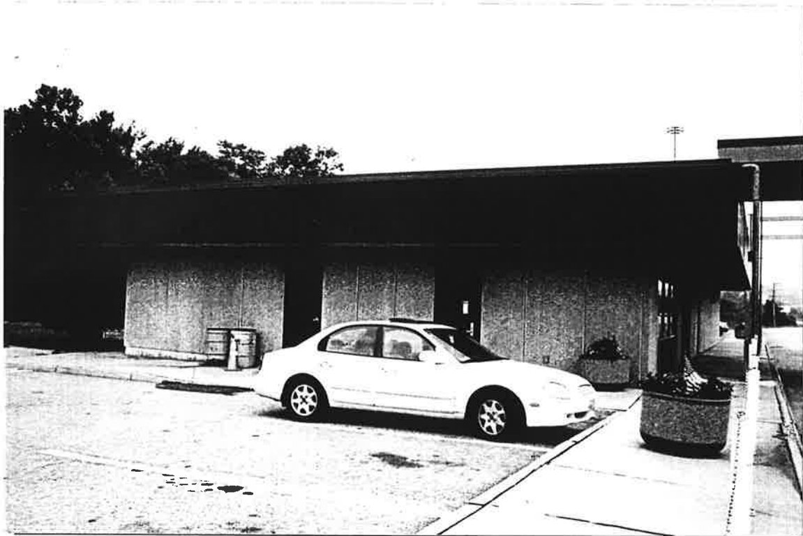
Photograph 3. East elevation, facing southwest.
