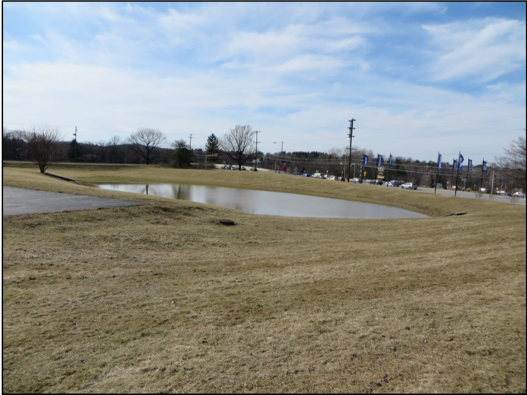
Photograph 9. Modern stormwater basin (ca. 1990) at the northwest corner of the campus, with the intersection of N. Gulph Road and 1 st Avenue in the background, view to northwest.
