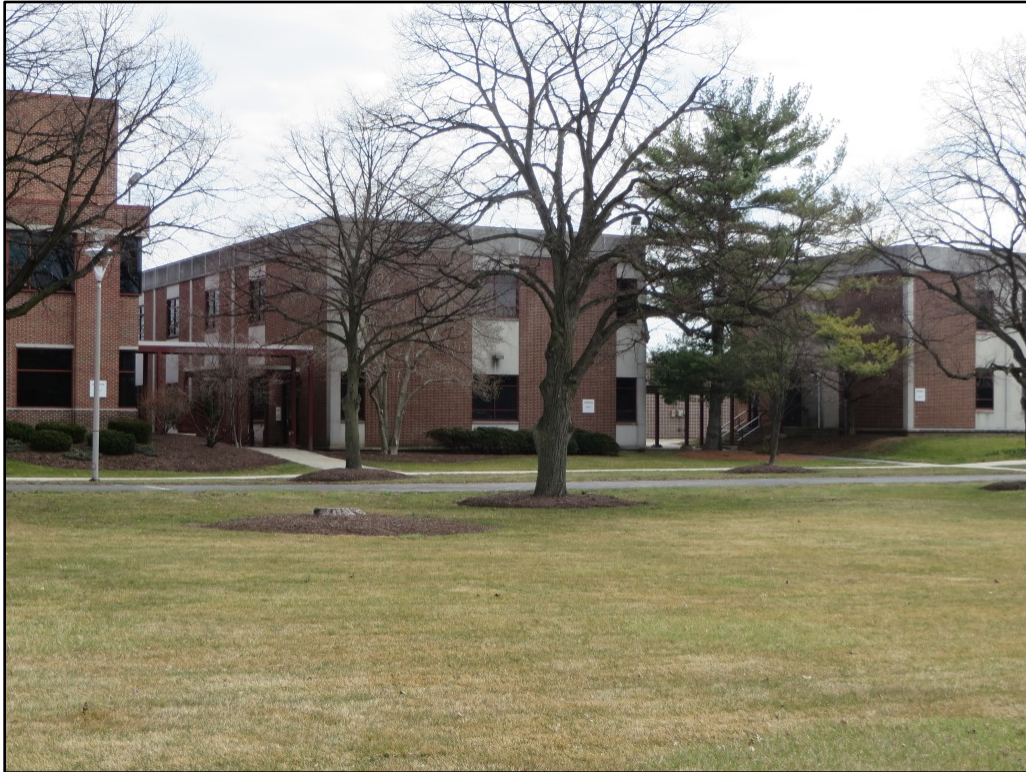
Photograph 13. View looking northeast showing the northwest (left) and southwest (center) elevations of Building 5 (ca. 1962), and covered passageways leading to Building 9 at left and Building 4 at right.
