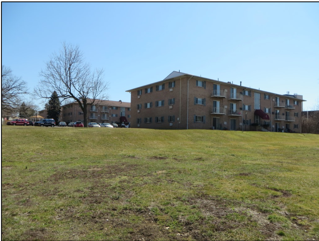
Photograph 4. View looking southeast toward King of Prussia Arms Apartments from Walker Field, with building C in foreground and building B at left rear.
