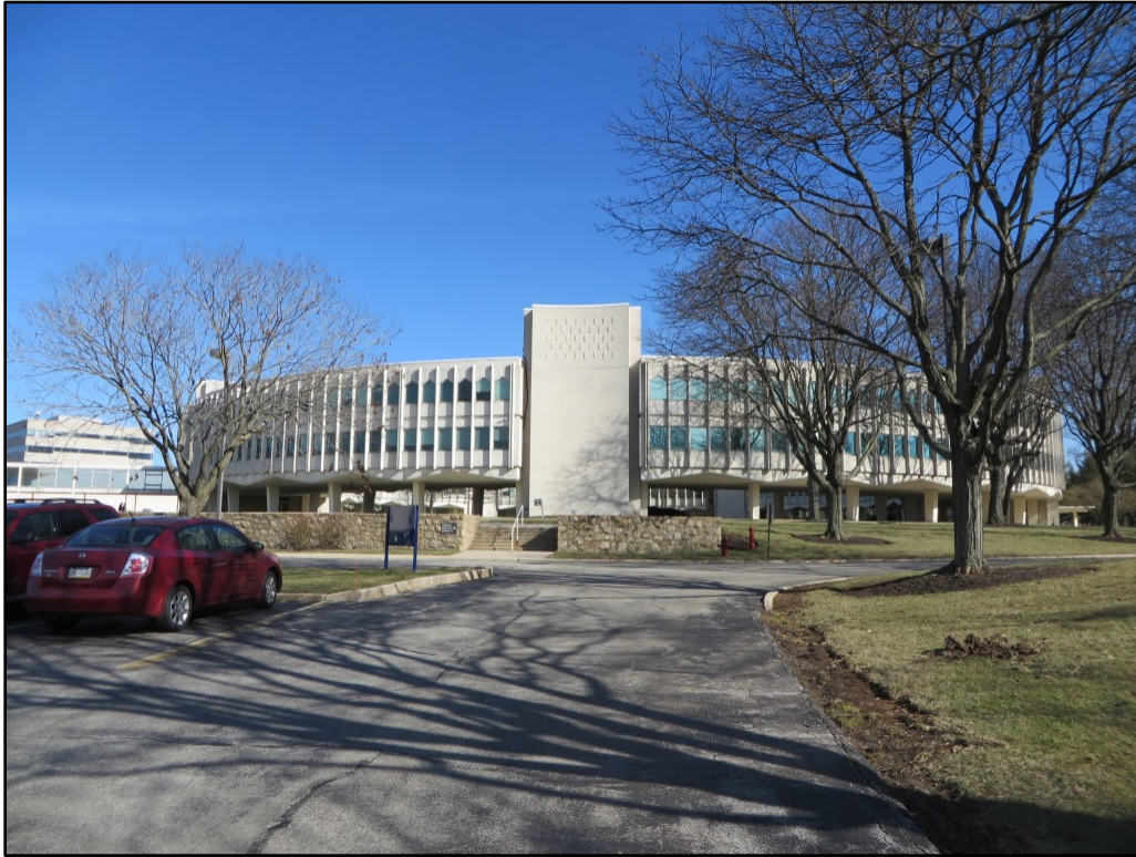
Photograph 13. View looking east toward the west exterior elevation of the Office and Conference Center; note open first floor space used as a covered walkway.
