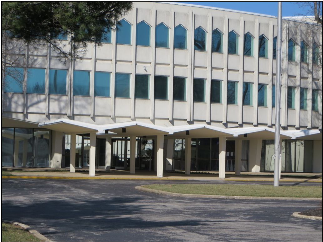
Photograph 18. Detail of the south-facing front entrance portico of the Office and Conference Center, view to northeast.
