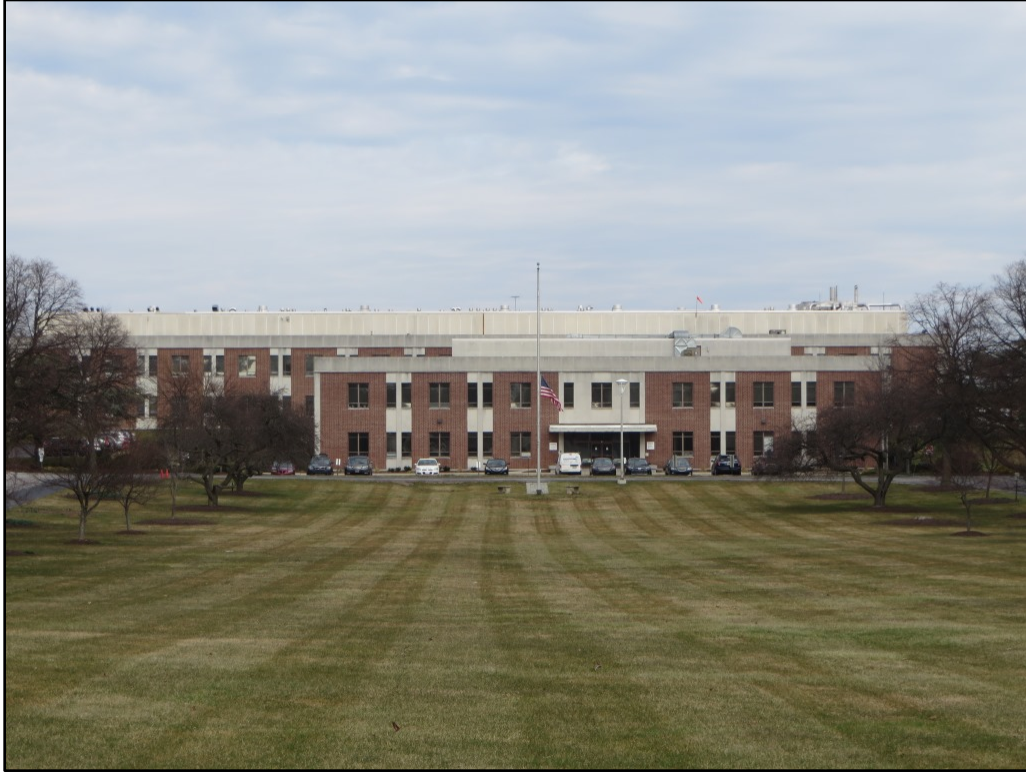
Photograph 9. View looking northwest showing Building 1 (ca. 1962) rising behind Building 2 (ca. 1962).
