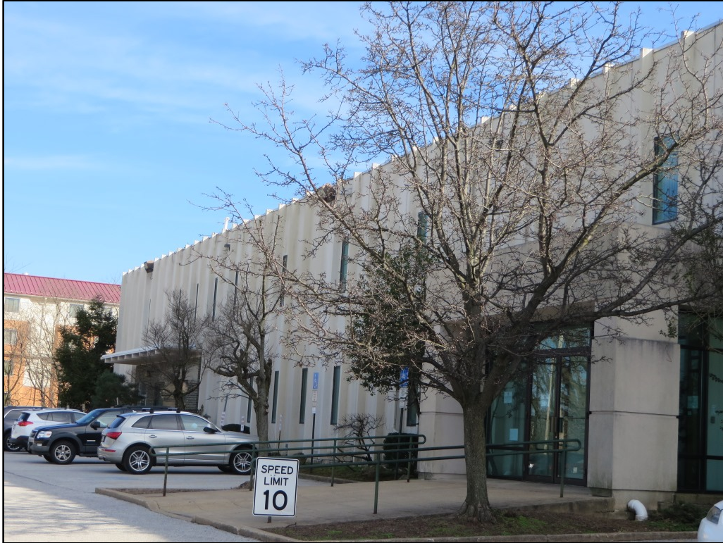
Photograph 3. View looking southeast toward the north elevation of the circa-1970 warehouse, showing the two front entrances.
