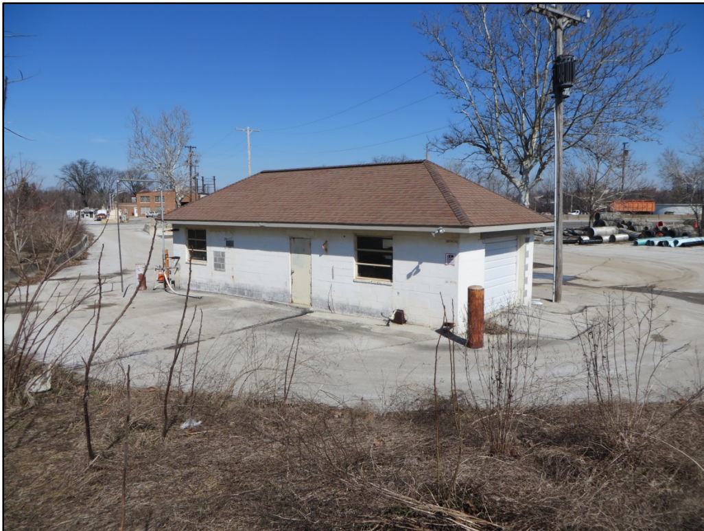
Photograph 8. View looking north from the southwest corner of the property with the circa-1975 pump house in foreground.
