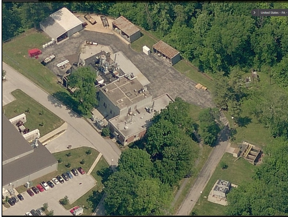
Bird's Eye View 3. Southwest (left) and southeast (right) elevations of Arkema Campus Pilot Plant complex with Building 3 at center, storage building and sheds at top, view to north (Bing 2016).
