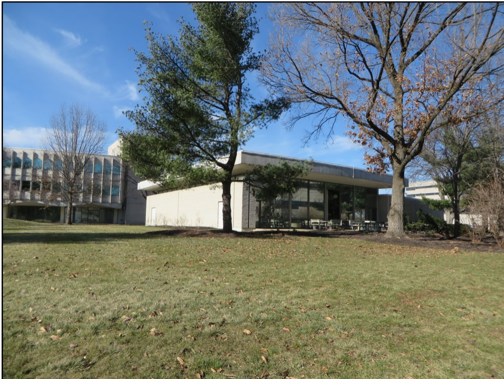
Photograph 22. Southwest (left) and southeast (right) elevations of the cafeteria, view to north. Note dining patio in front of the southeast elevation and shorter kitchen wing to the right.
