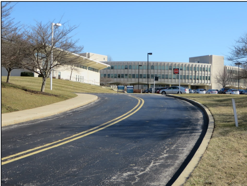
Photograph 6. View looking southeast up the north driveway from 1 st Avenue, showing the Graphic Arts Building at left and the Office and Conference Center at center and right.
