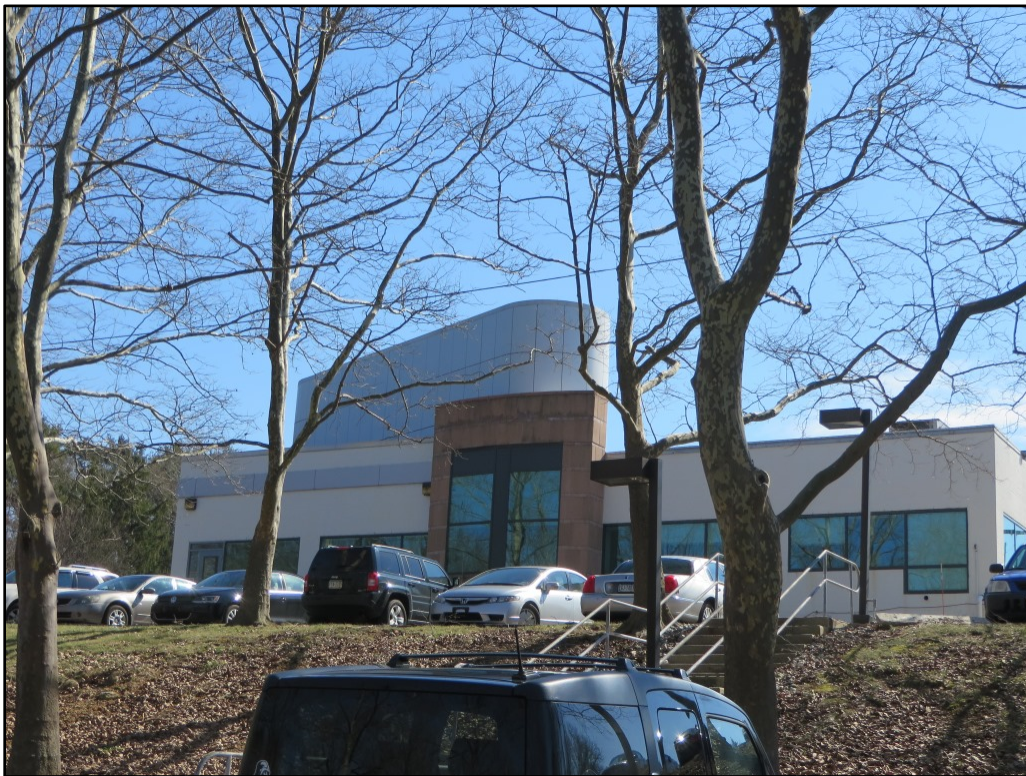
Photograph 4. North elevation of the circa-1964 building, looking southeast. Façade treatments date from an extensive remodeling ca. 1980.
