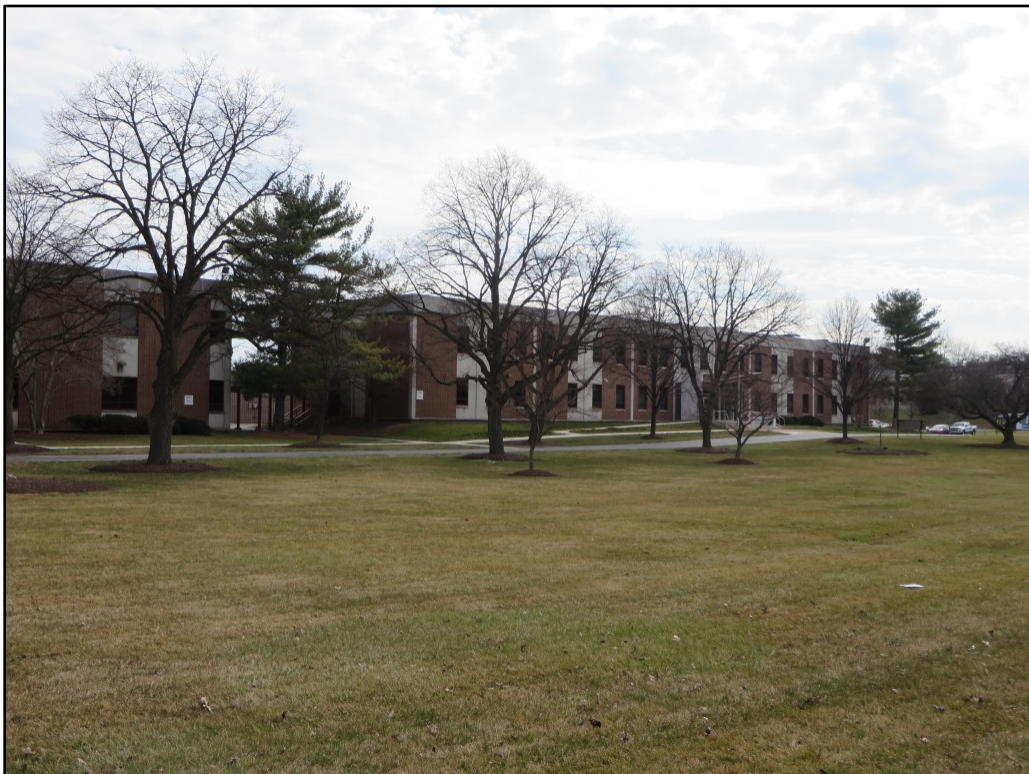
Photograph 12. View looking east toward the southeast elevations of Building 5 (ca. 1962) at left and Building 4 (ca. 1960) at center-right.
