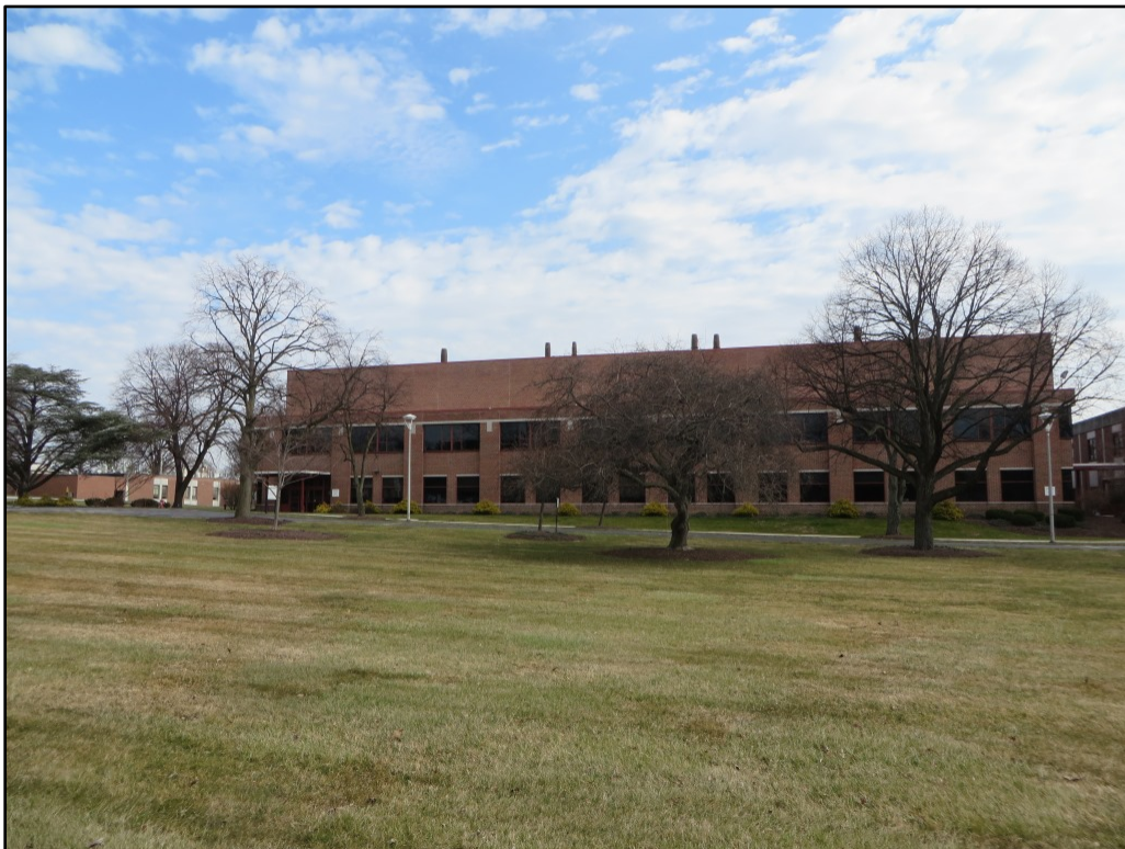
Photograph 16. View looking northeast toward the southwest elevation of Building 9. Building 6 is visible in left background.
