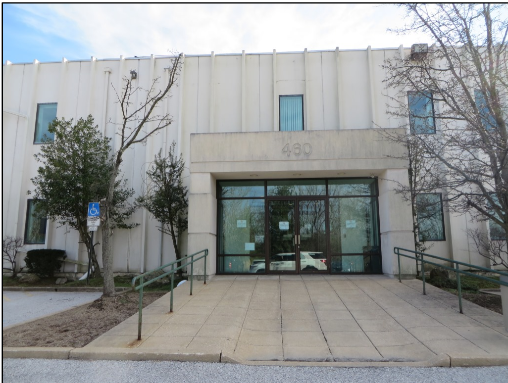
Photograph 4. View looking south toward the main (center) entrance in the north elevation of the circa-1970 warehouse.
