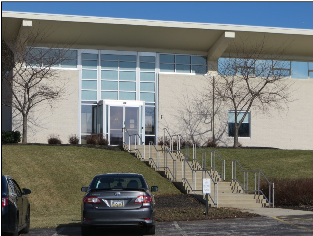
Photograph 26. Detail view looking northeast toward the modernized west elevation entrance of the Graphic Arts Building. Original clerestory windows are located at upper right.
