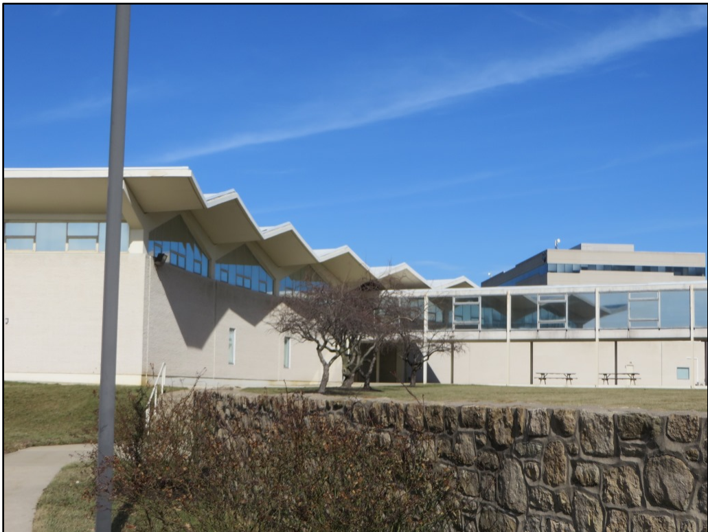
Photograph 24. West (left) and south (inner) elevations of the Graphic Arts Building, with two-story west hyphen at right connecting it to the Office and Conference Center; view to northeast.
