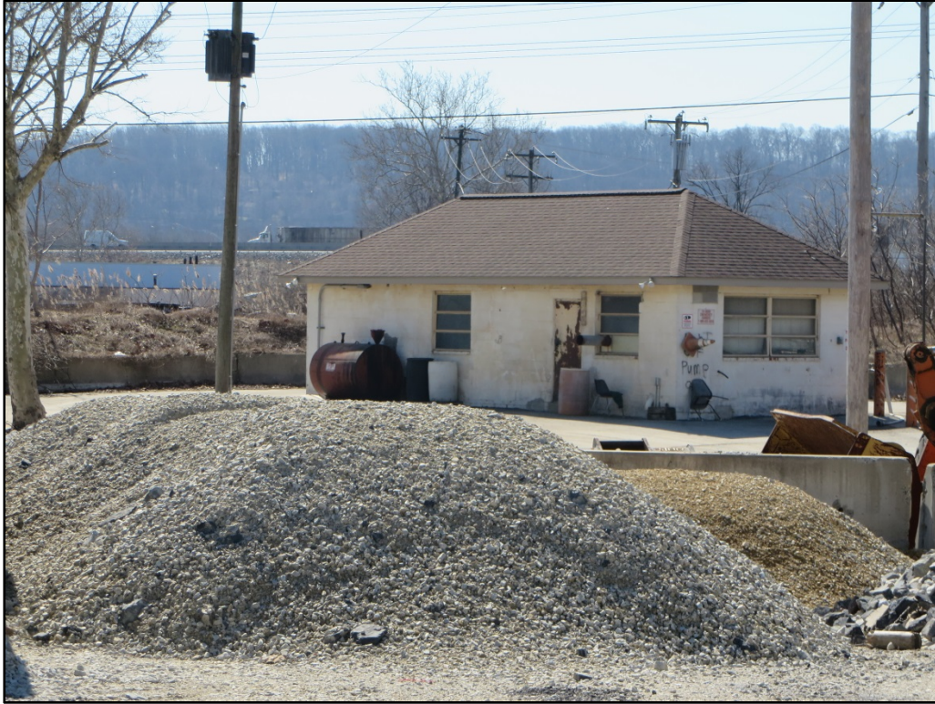
Photograph 7. View looking southwest toward the circa-1975 pump house.
