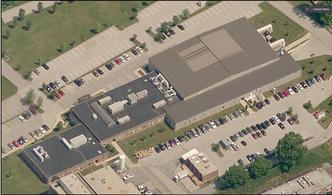
Bird's Eye View 11. Southwest (left) and southeast (right) elevations of Arkema Campus Buildings 12 (left) and 14 (right), view to north. Building 7 is in the lower foreground (Bing 2016).
