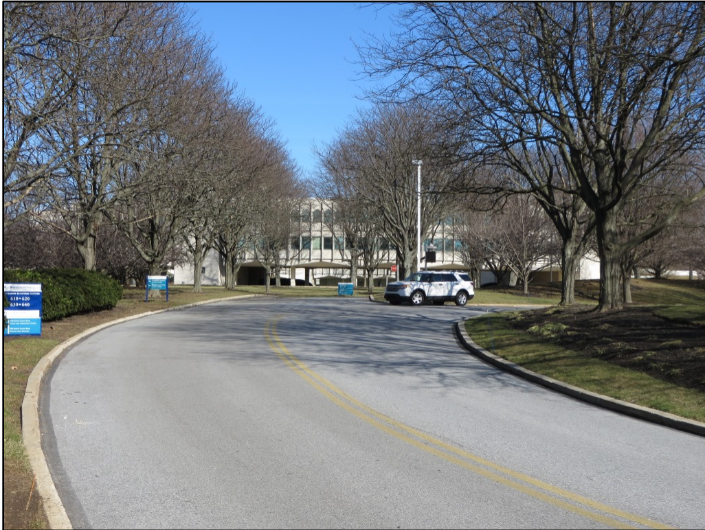
Photograph 1. West driveway entrance (Freedom Business Center Drive) off N. Gulph Road into the ABCUSA Mission Center complex, looking east toward the Office and Conference Center (ca. 1962).
