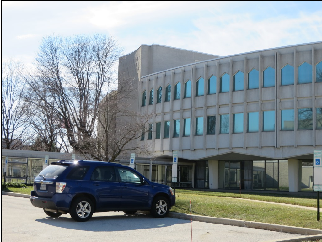
Photograph 15. View looking southwest toward the southeast exterior elevation of the Office and Conference Center, with original hyphen connecting it to the cafeteria building at left and center.
