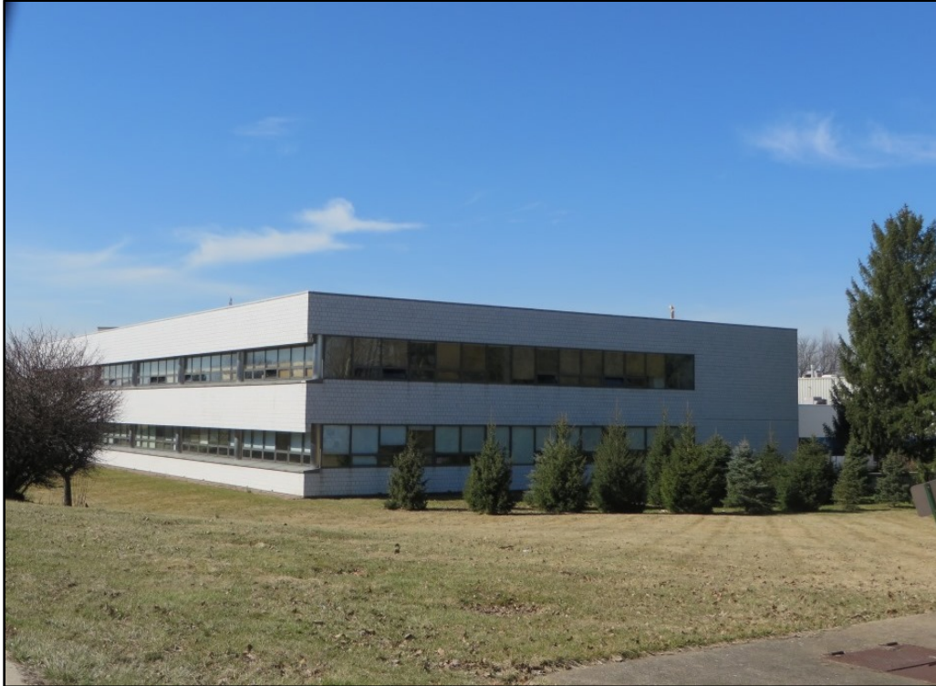
Photograph 7. South (left) and east (right) elevations of the circa-1964 building; façade treatments date from an addition to the south front and extensive remodeling ca. 1980.
