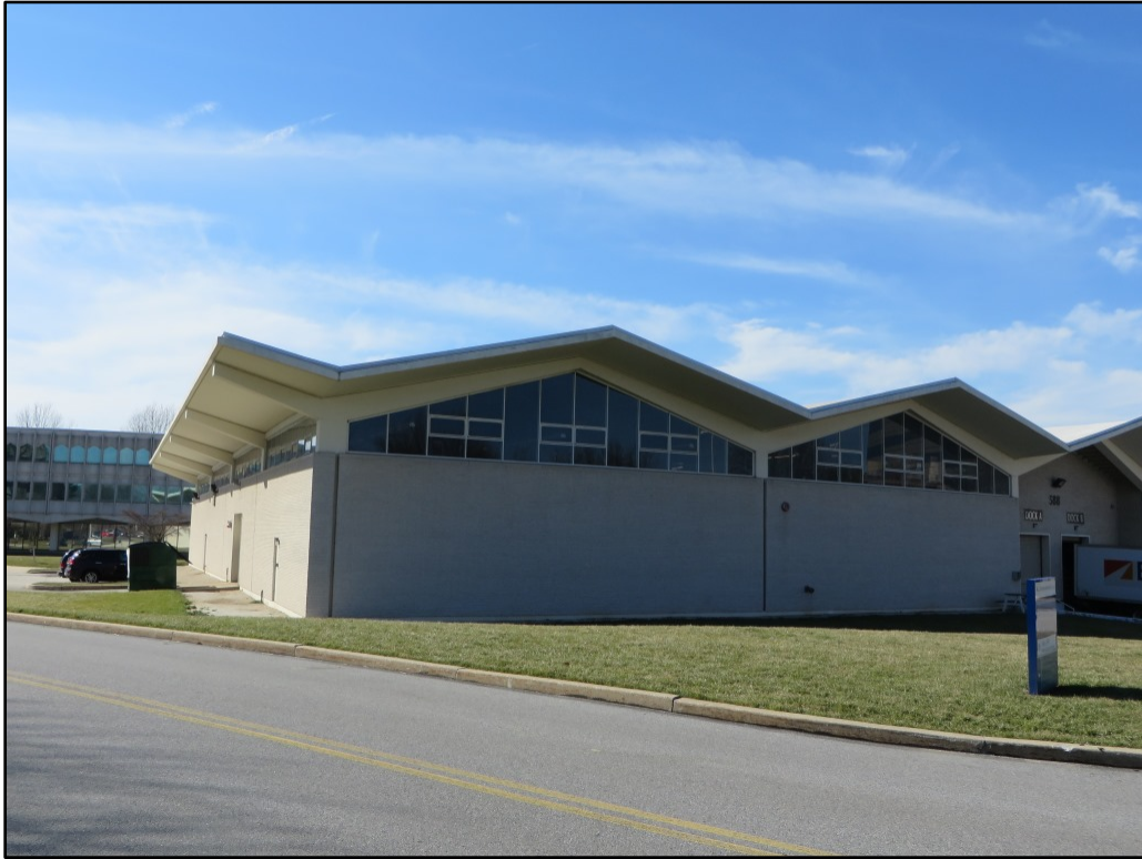
Photograph 29. South elevation (left) and east side of the outer elevation (right) of the Graphic Arts Building, view to west. Second loading dock is at right.
