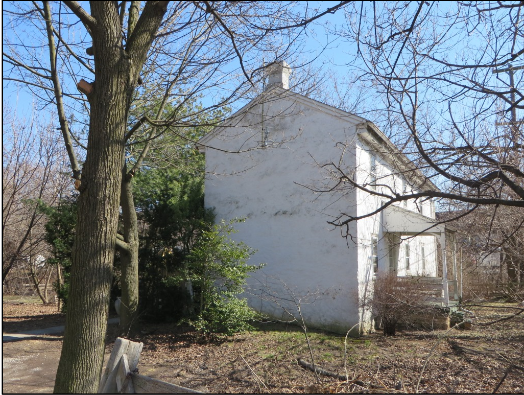
Photograph 3. View looking southeast toward the northwest (center) and southwest (right) elevations of the circa-1860 dwelling.
