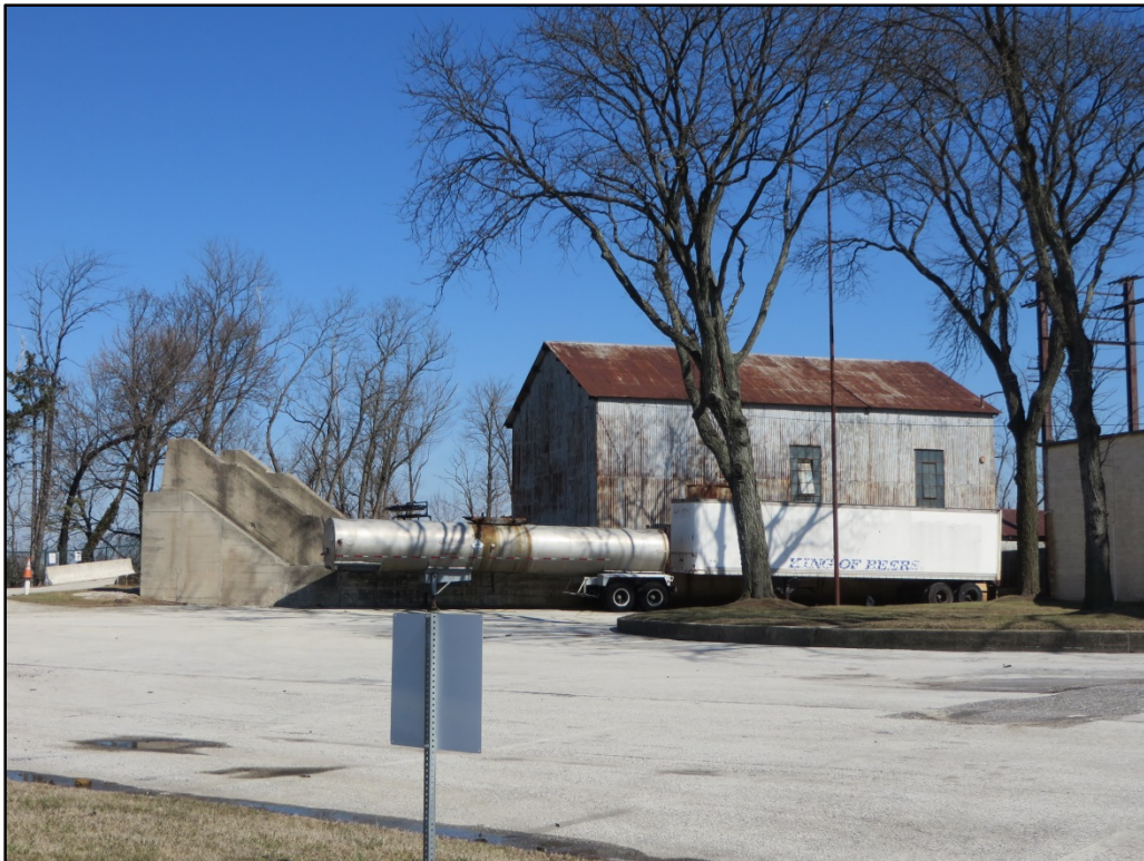
Photograph 10. View looking northeast toward the west (left) and south (right) elevations of the circa-1940 metal quarry shed.
