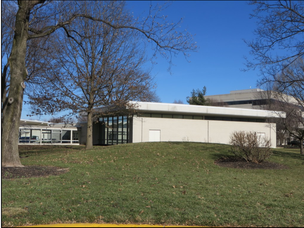
Photograph 21. View looking northeast toward the northwest (left) and southwest (right) elevations of the cafeteria (ca. 1962). Note connecting hyphen at left.
