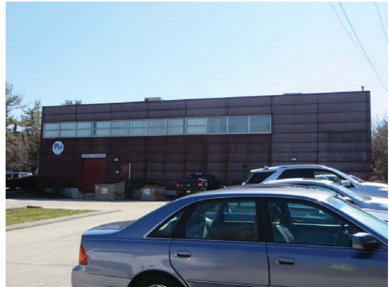
Caption: Photograph 2. North elevation of circa-1970 building, view to southeast.
