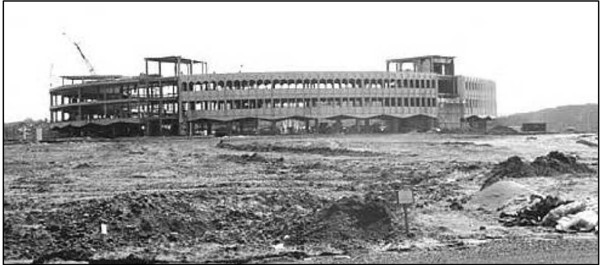
Figure 7. Photo of the Office and Conference Center during construction ca. 1961 (Laubach 2010:34).
