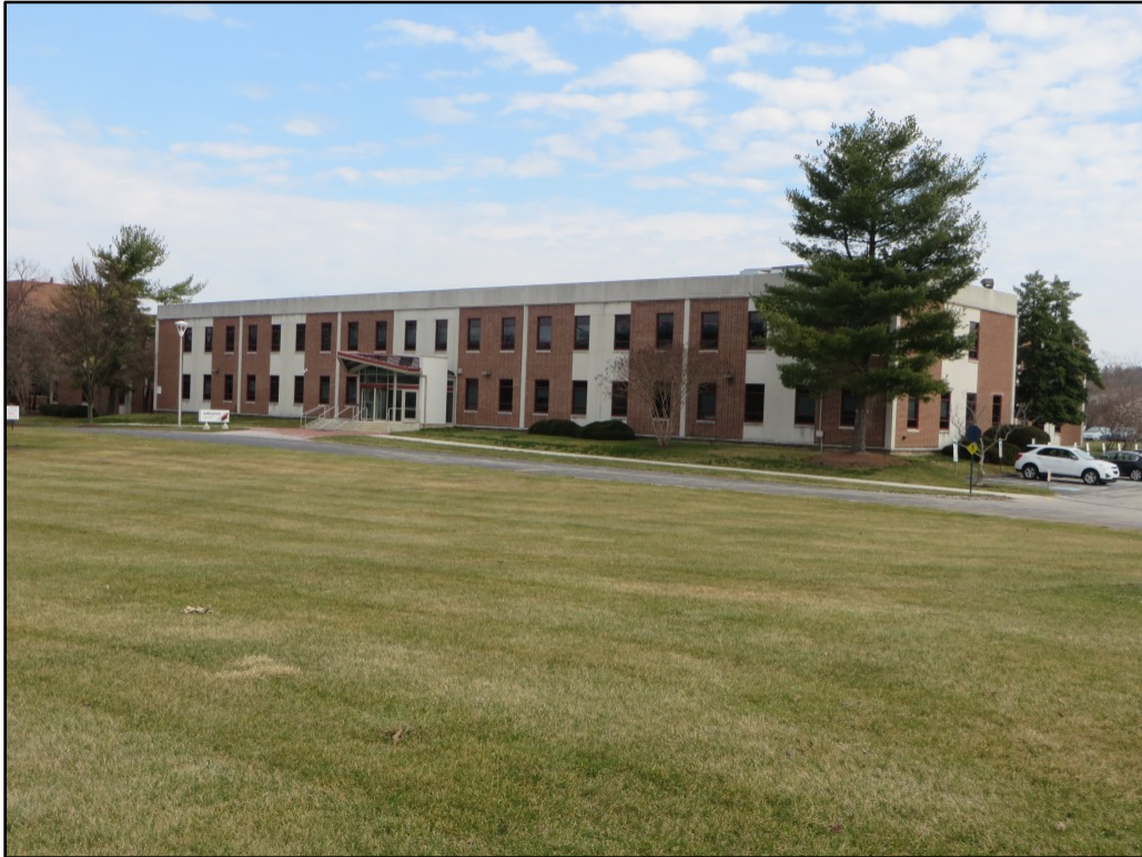
Photograph 11. View looking northeast toward the southwest (left) and southeast (right) elevations of Building 4 (ca. 1960). Building 4 was renovated in recent years and now houses a secondary lobby for the campus.
