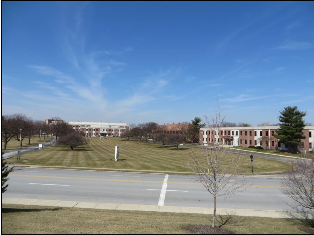
Photograph 1. General view looking north across First Avenue toward the Arkema Campus. Note the front mall arrangement and dual driveways; West Driveway is at left and Center Driveway at right.
