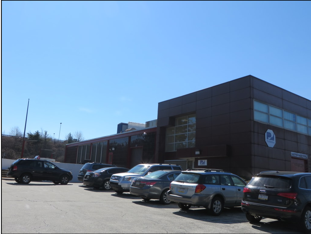
Photograph 3. East (center) and north (right) elevations of the circa 1970 building.
