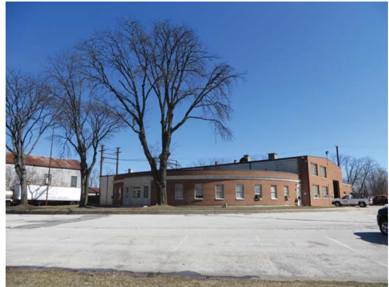
Caption: Photograph 2. View looking northeast toward west elevation of main building (ca. 1940) with semicircular front addition (ca. 1965).
