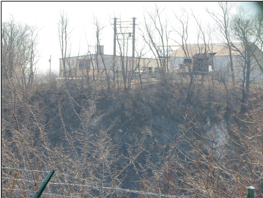
Photograph 12. View looking southeast across the McCoy Quarry pit from its northwest corner toward the building complex, with the circa-1940 main building at left and the circa-1940 quarry shed at right.
