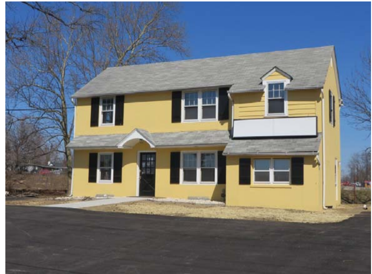
Caption: Photograph 2. Southwest (center) and northeast (right) elevations of the circa-1945 dwelling, view to northeast.
