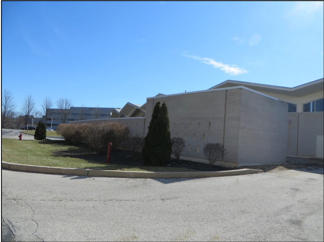
Photograph 31. Enclosed original utility area on the northwest side of the Graphic Arts Building, with ornamental pierced brick walls; view to south.
