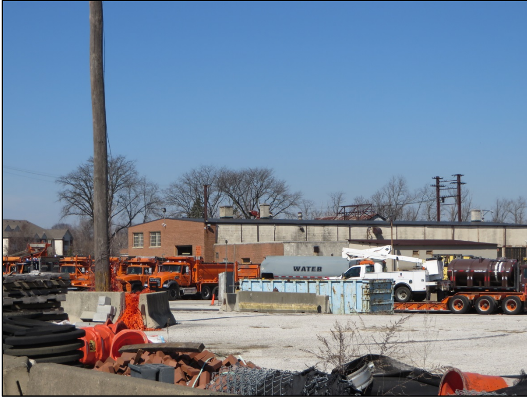
Photograph 5. View looking northwest from east side of property toward the south (left) and east (right) elevations of the circa-1940 main building.
