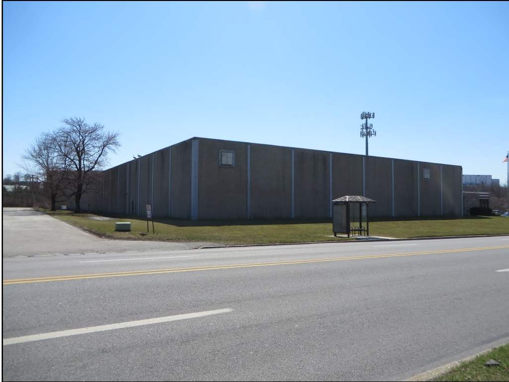
Photograph 3. View looking south toward the northeast (left) and northwest (right) elevations of the circa-1965 warehouse.
