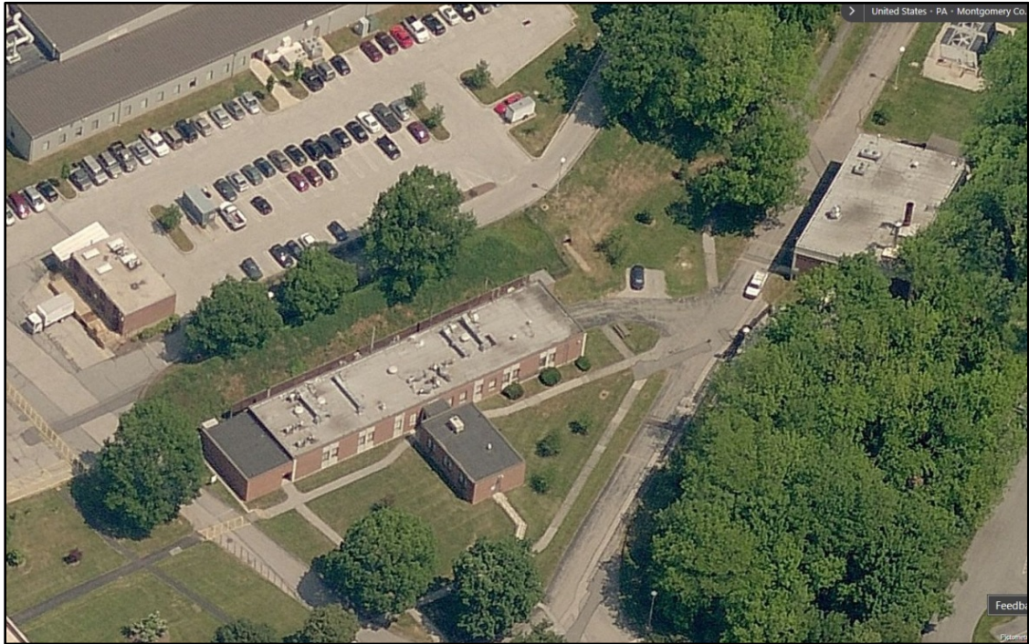
Bird's Eye View 9. Southwest (left) and southeast (right) elevations of Arkema Campus Buildings 6 (center), 7 (upper left), and 8 (upper right), view to north. Note modern additions to the southwest and southeast elevations of Building 6 (Bing 2016).
