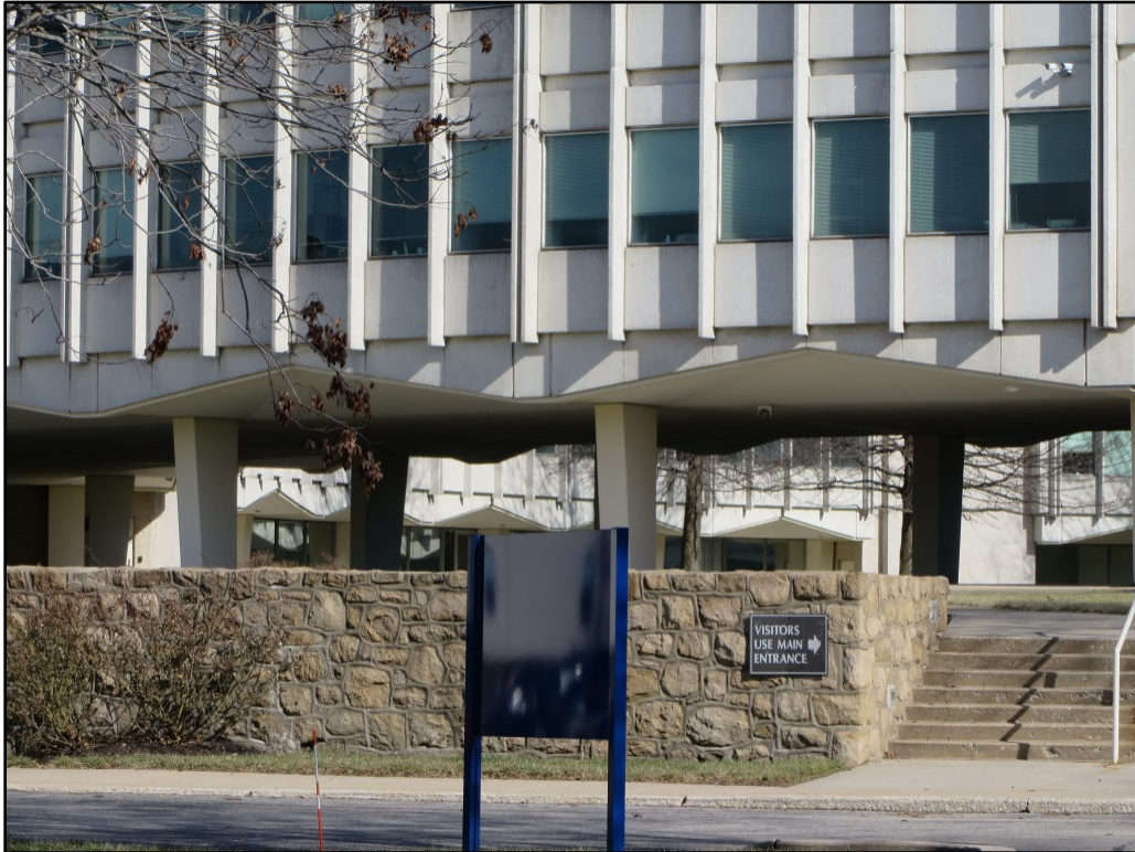
Photograph 11. Original stone retaining wall, concrete steps, and sidewalks along the west side of the Office and Conference Center, view to east.
