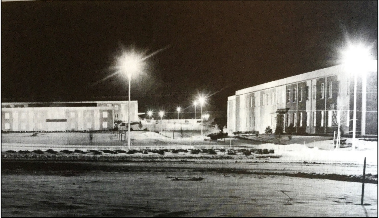
Figure 7. 1963 view of Buildings 1 and 2 at left, and Building 4 at right at the newly completed Pennsalt Technological Center. This photo appeared in the 1963 Pennsalt annual report (Pennsalt Chemicals Corporation 1964).
