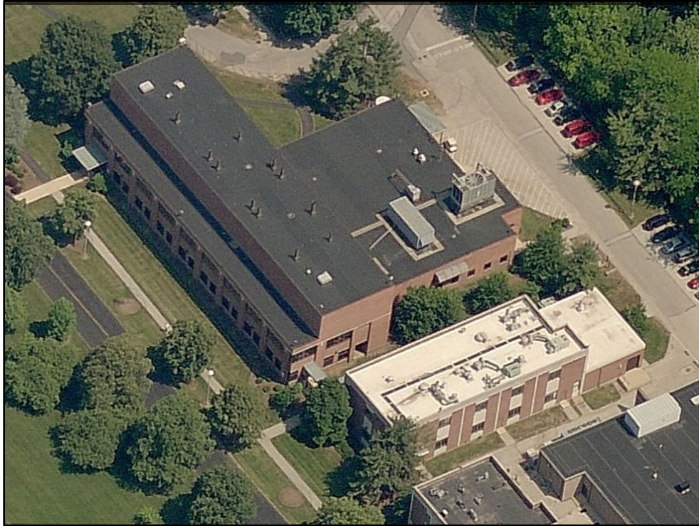
Bird's Eye View 7. Southwest (left) and southeast (right) elevations of Arkema Campus Buildings 5 (bottom) and 9 (top), view to north (Bing 2016).
