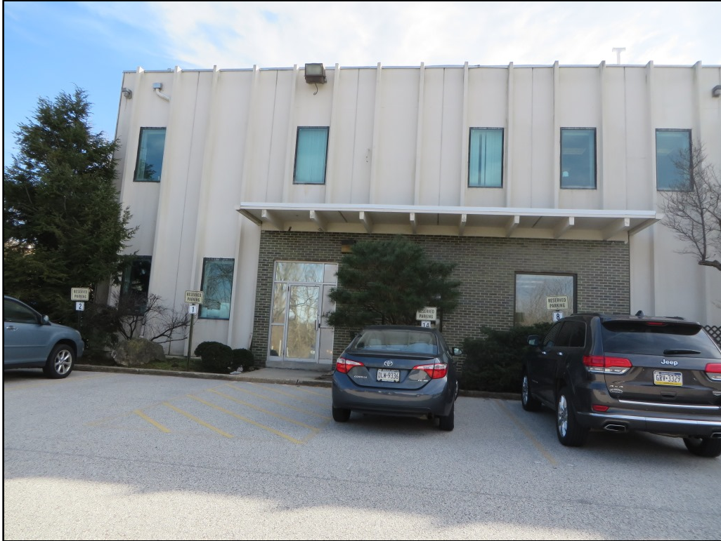
Photograph 5. View looking south toward the secondary (east) entrance in the north elevation of the circa-1970 warehouse.
