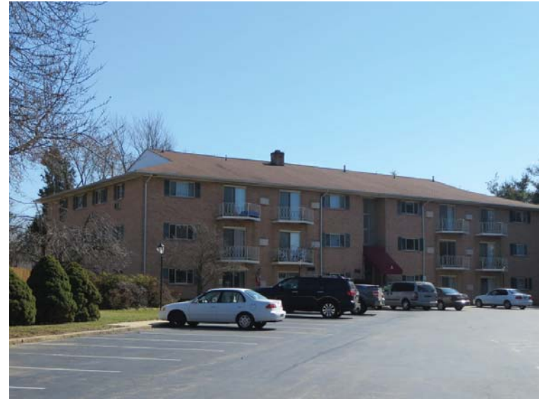
Caption: Photograph 1. North (left) and west (center) elevations of the circa-1962 apartment building A, view to southeast.
