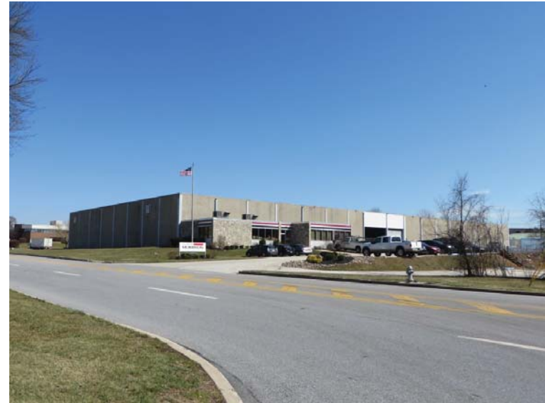
Caption: Photograph 1. Northwest (left) and southwest (right) elevations of circa 1965 warehouse building, view to east.
