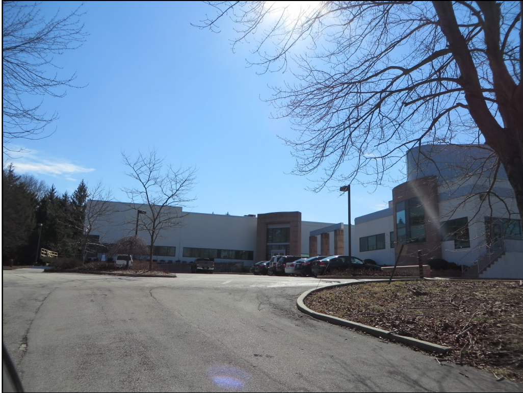
Photograph 5. North (left) and east (right) elevations of the circa-1964 building, view to southwest. Façade treatments date from an extensive remodeling ca. 1980.
