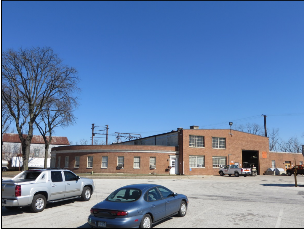
Photograph 3. View looking northeast toward west (left) and south (right) elevations of main building, with additions (ca. 1965) on left and right of the 2-story circa-1940 main block.
