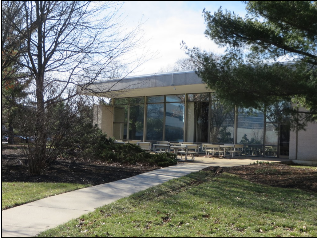
Photograph 23. Southeast elevation of the cafeteria and dining patio, view to west.
