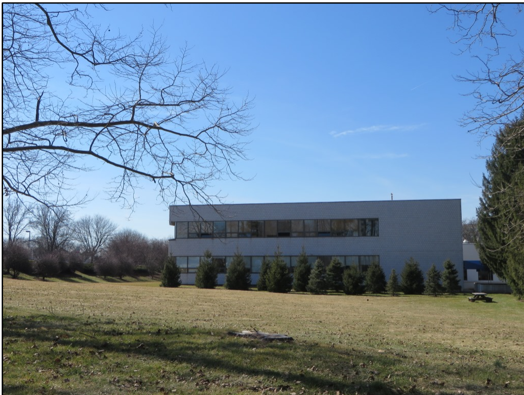
Photograph 6. East elevation of the circa-1964 building; façade treatments date from an addition to the south front and extensive remodeling ca. 1980.
