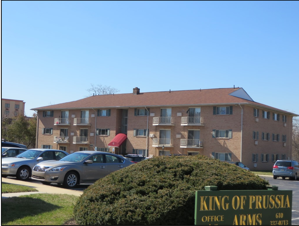
Photograph 3. View looking southwest toward the east (center) and north (right) elevations of the circa-1962 apartment building C in the King of Prussia Arms Apartments.
