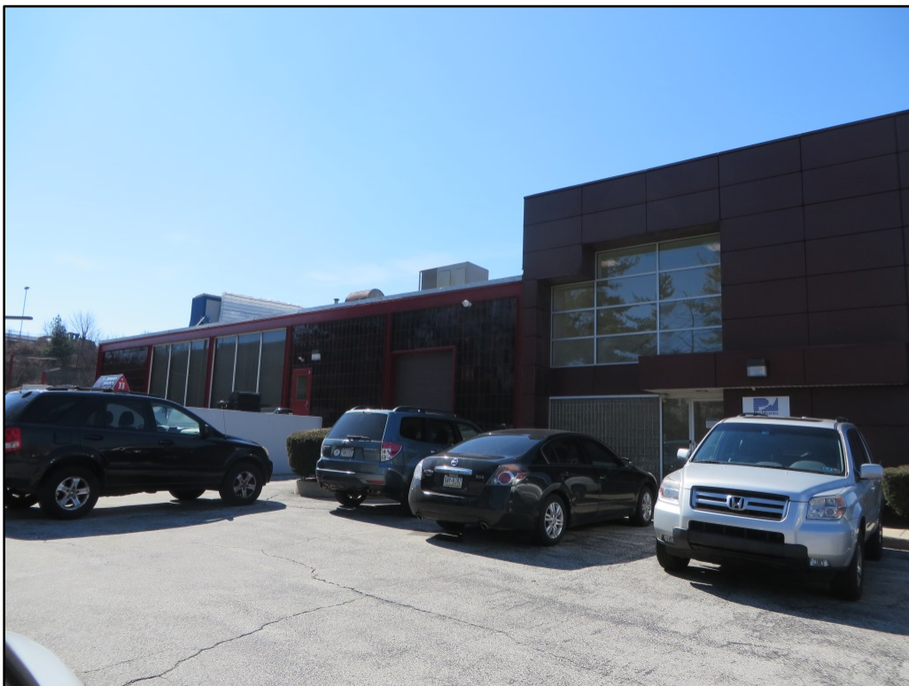
Photograph 4. Detail view of loading dock and entrance in east elevation of the circa-1970 building; note ceramic tile exterior cladding.
