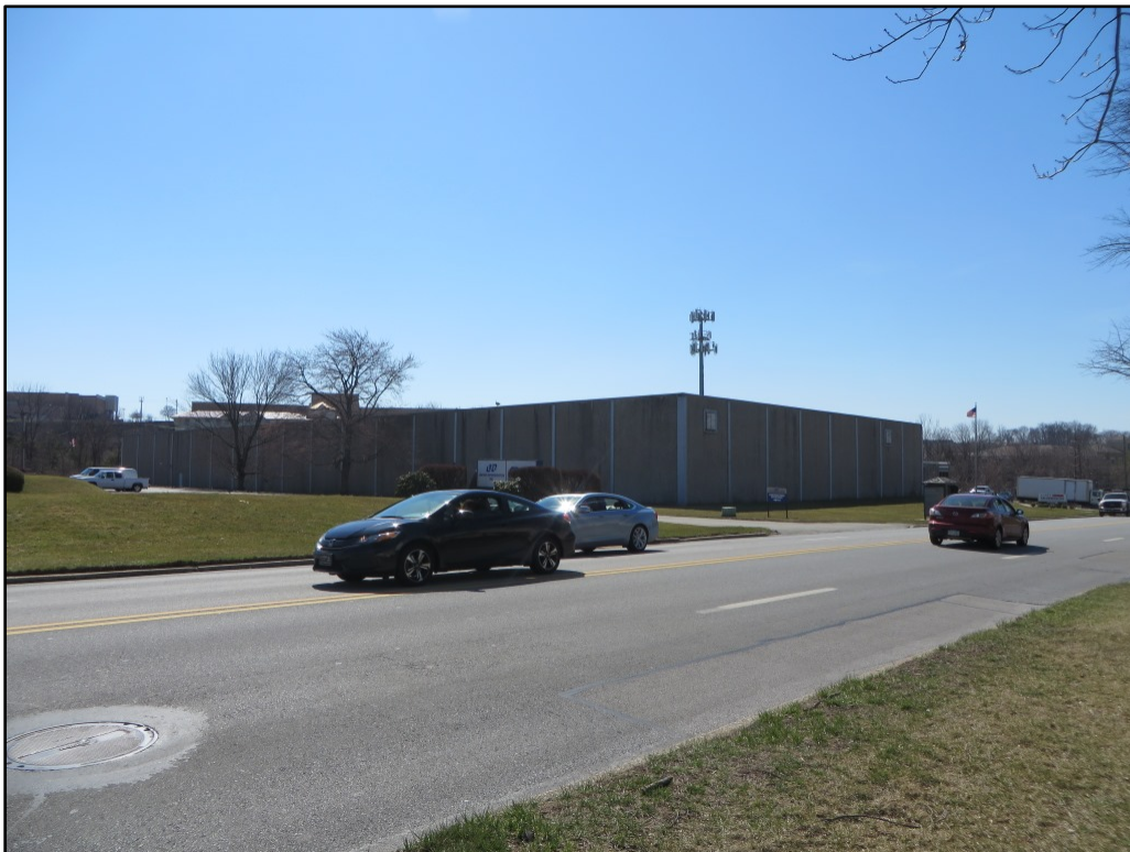
Photograph 4. View looking southwest toward the northeast (left) and northwest (right) elevations of the circa-1965 warehouse.
