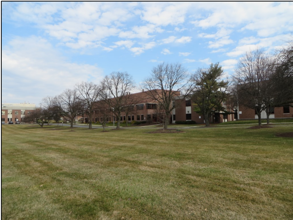
Photograph 14. View looking north showing Building 2 at far left, Building 9 (ca. 1991) at center, and Buildings 5 and 4 at right. The location of Building 9 was originally an open lawn area.
