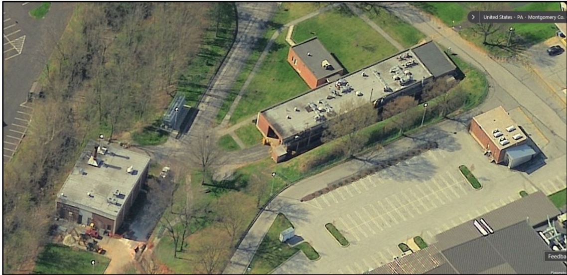
Bird's Eye View 10. Northeast (left) and northwest (right) elevations of Arkema Campus Buildings 6 (center), 7 (right), and 8 (left), view to south (Bing 2016).
