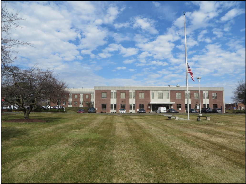
Photograph 7. Southeast elevations of Building 1 (background, left) and Building 2 (center right), view looking north from the mall. Building 2 contains the primary lobby for the campus.
