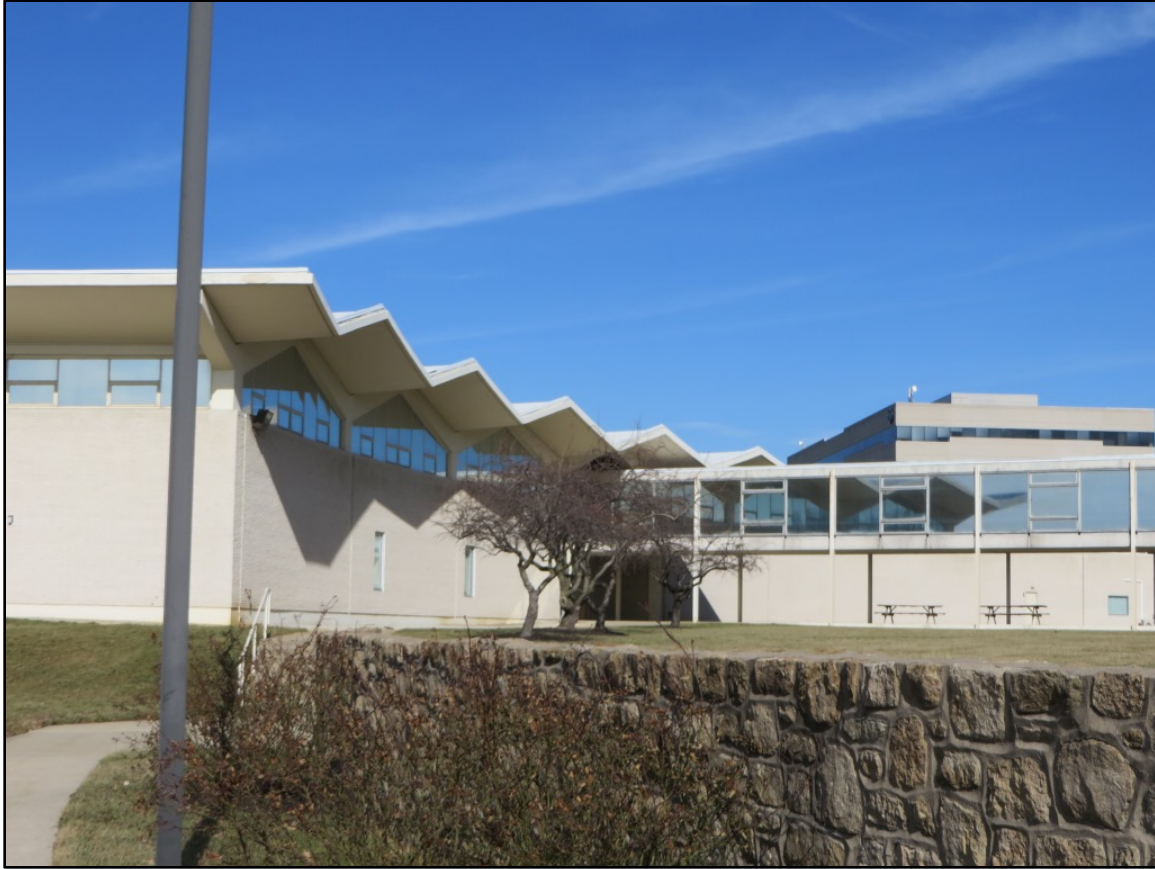
Photograph 2. View of the Graphic Arts Building, looking northeast.
