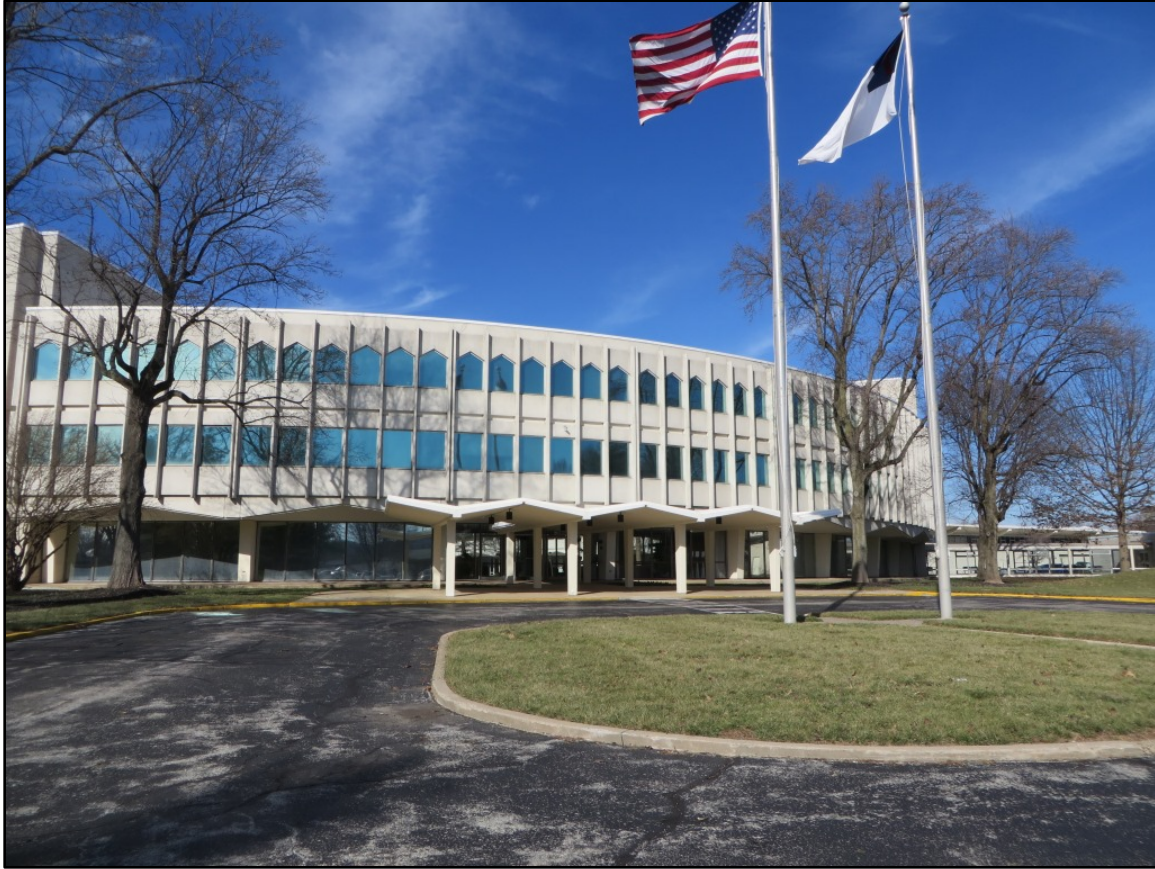
Photograph 1. South elevation of the Office and Conference Center building, view to east.
